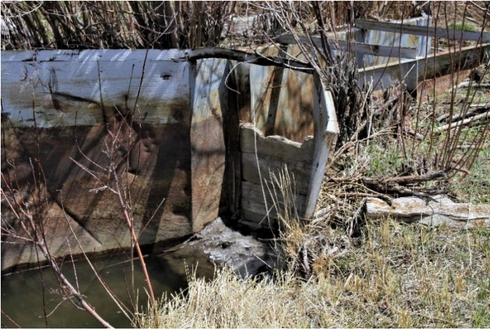
Headgate looking downstream
