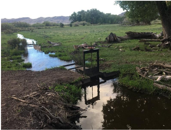
Headgate looking downstream
