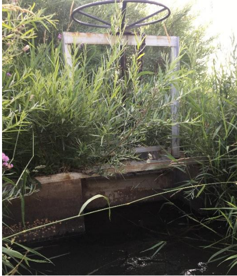
Headgate looking downstream
