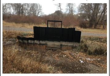
Ditch carrier made of corrugated plastic pipe
