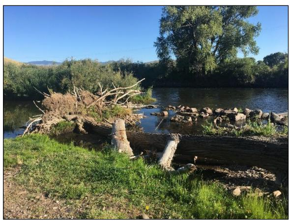
Point of diversion, post-2019 runoff. This cottonwood is currently blocking the feeder channel.
