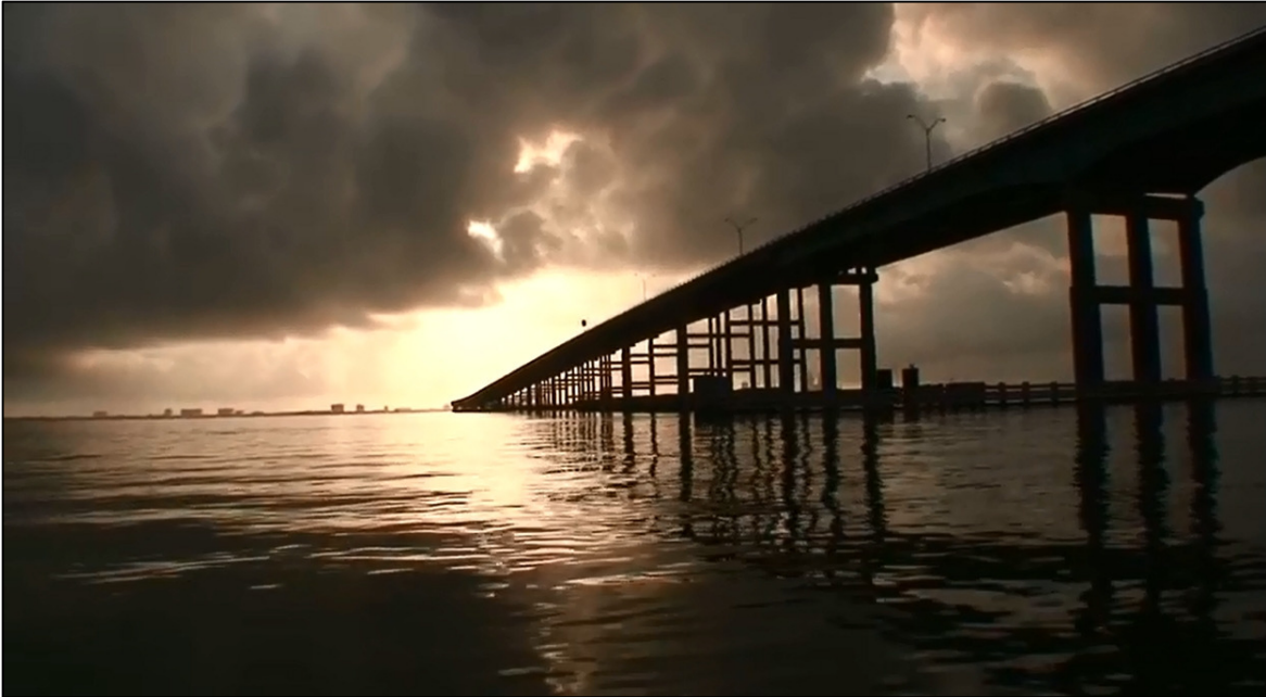
Storm clouds over the Gulf as we headed toward the inlet
