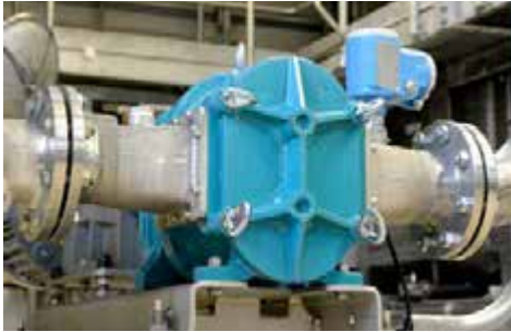
BLUEline pump for conveying cleaning agents
