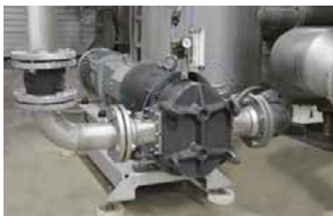
ONIXline pump for conveying Starch Slurry
