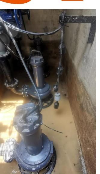
Tsurumi installed 3 units of MYB550 for a detention tank at an industrial factory on the West Coast of Singapore.
