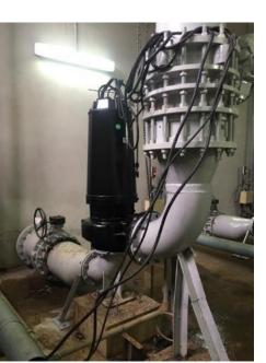
The MQ-series pump incorporates an IE3 premium efficiency motor to enhance its overall performance and energy efficiency. With the addition of the cooling jacket, the pump is capable of effectively dissipating heat during operation, ensuring its longevity and reliability in demanding conditions.
