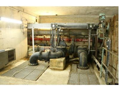
A single unit of the TSURUMI AVANT pump, model MQB 300C 37/6AW 370, has been successfully installed at a sewage pumping station located at a metro depot in Hong Kong.
