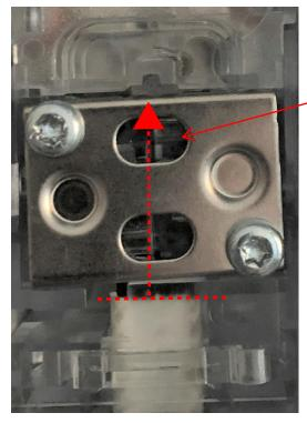
The heating cable inner jacket should be visible in both windows
