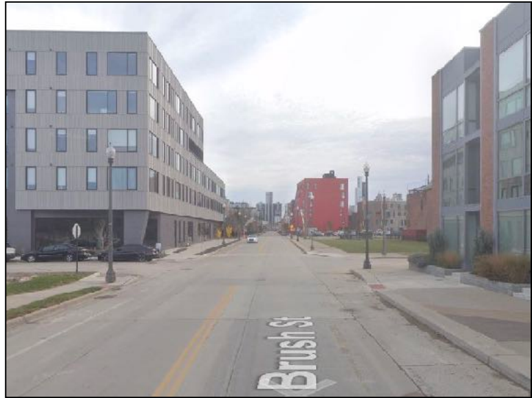
Southern facing view of Brush St & Watson intersection
