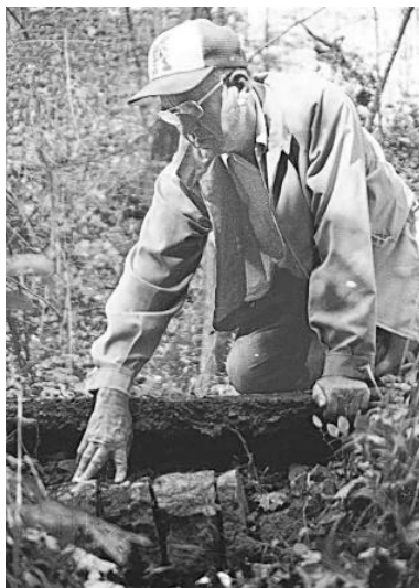
West Point historian Richard Briggs examines a portion of the macadamized roadbed of the old Louisville and Nashville turnpike, beneath the modern asphalt surface, at the Bridges to the Past walking trail. – Photo by Paul W. Urbahns
