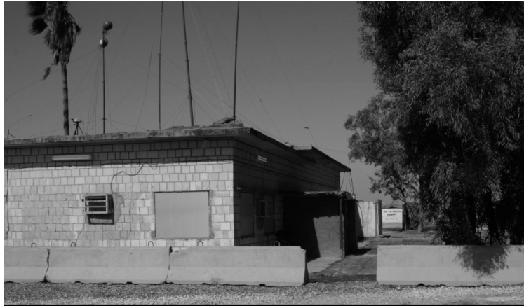
1st Battalion 158th Field Artillery Headquarters Building Camp Ramadi
