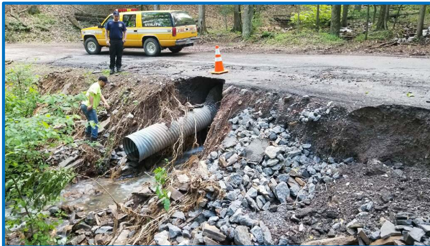
Figure 4.3.8-6: Emergency Management crews respond to a collapsed portion of Bowers Lane in Morgan County (Morgan County EM)
