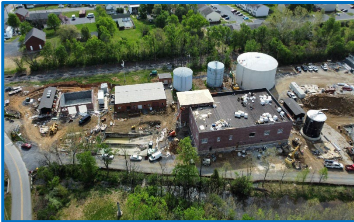
Figure 4.3.20-1 The New Bunker Hill Plant Under Construction as of April 2026 (BCPSWD, 2026a).
