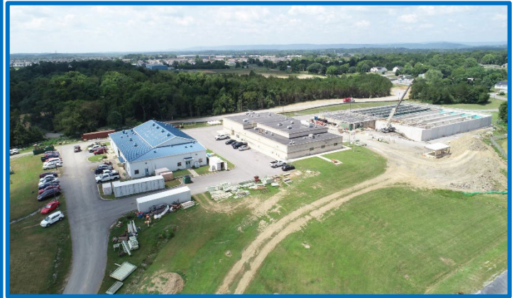
Figure 4.3.20-2 The Potomac River Plant Expansion Progress as of July 2025 (BCPSWD, 2025).
