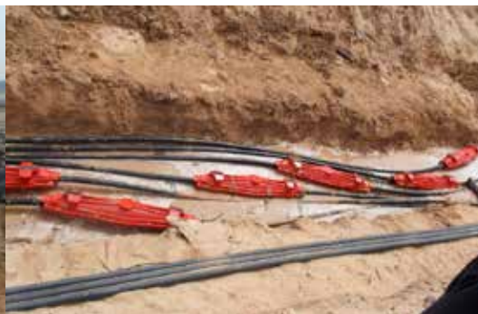
Straight through joints high water table
