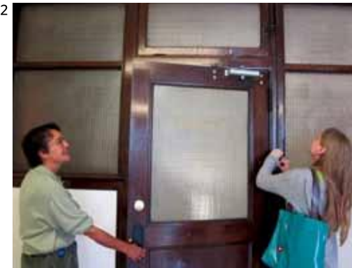
40 Recommended: [42] Transoms and screen doors are distinctive and practical features that provided cross ventilation in this historic hotel.
