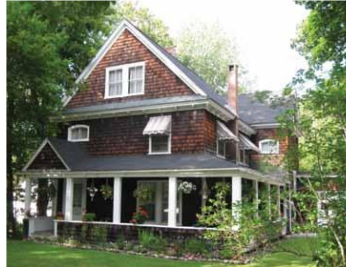
41 Recommended: [41] Traditional canvas awnings should be retained when they exist on historic buildings.
