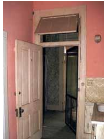
42 Recommended: [43] The wall and door glazing ensures that the corridor receives natural daylight and the operable transom helps air to circulate in this historic office building.
