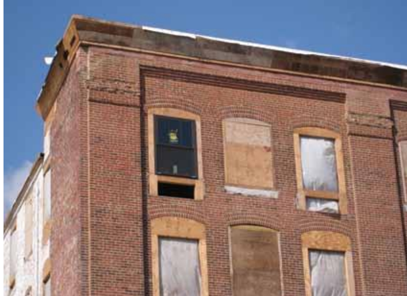
Not Recommended: [30] Not only have incompatible windows that do not fit the size and shape of the historic window openings been installed, but the original openings have also been shortened to install through-the-wall HVAC units.
