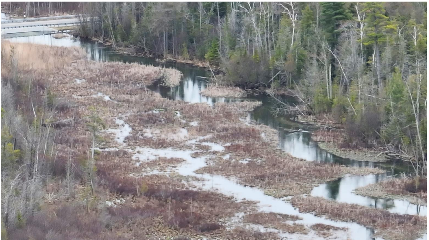
Eastward view downstream of 669 Bridge, note the flat gradual slope and standing water up to 669 Bridge
