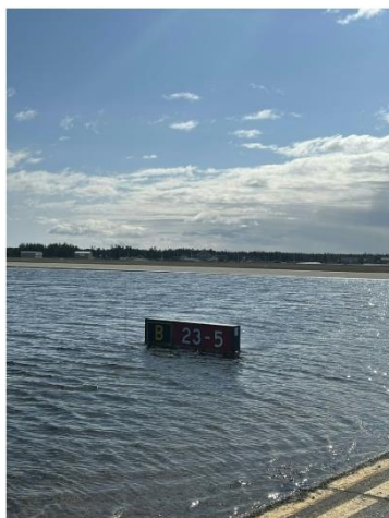
Flooded areas at the Pellston Regional Airport. Photo courtesy of the Pellston Regional Airport
