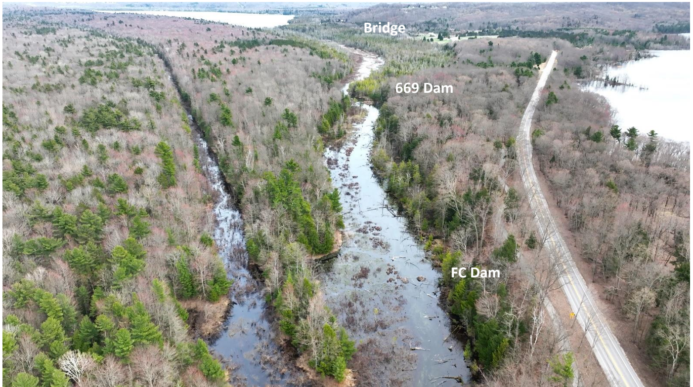
Eastward view towards LTL from Y intersection of Shalda Creek (right) and Juniper Drain (left) Locations of Bridge ("B"), 669 Dam ("669") and Fish Camp Dam ("FC" noted)
