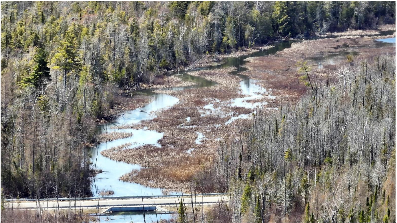
Westward view downstream of 669 Bridge, note the flat gradual slope and standing water
