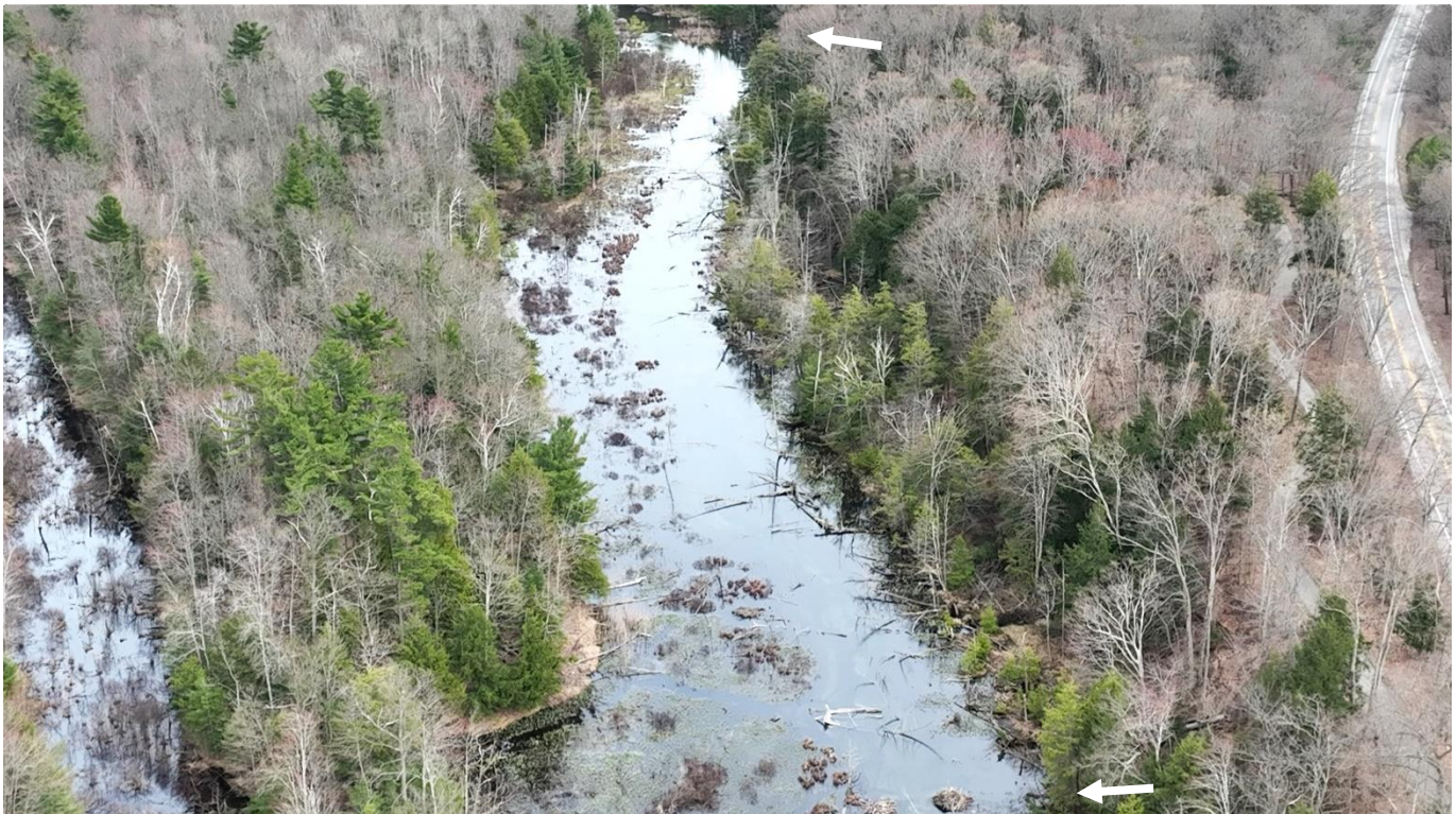
Closer view of section between Fish Camp Dam (bottom downstream) and 669 Dam (top, upstream)
