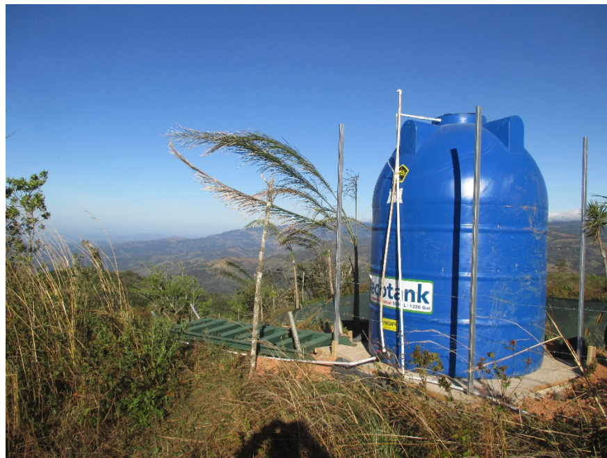
5,000 Liter Tank now installed for Potable Water System
