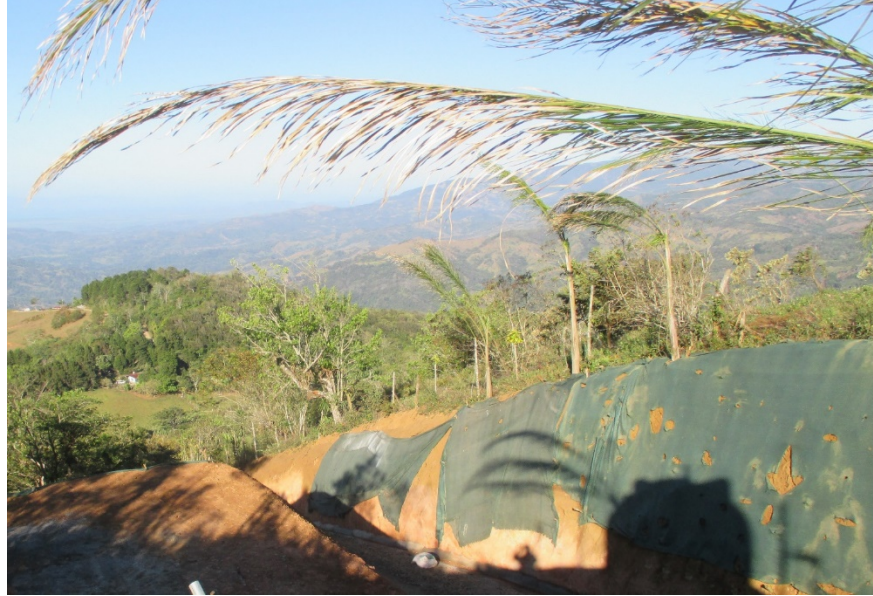
Curb and Gutter will be finished by mid-February
