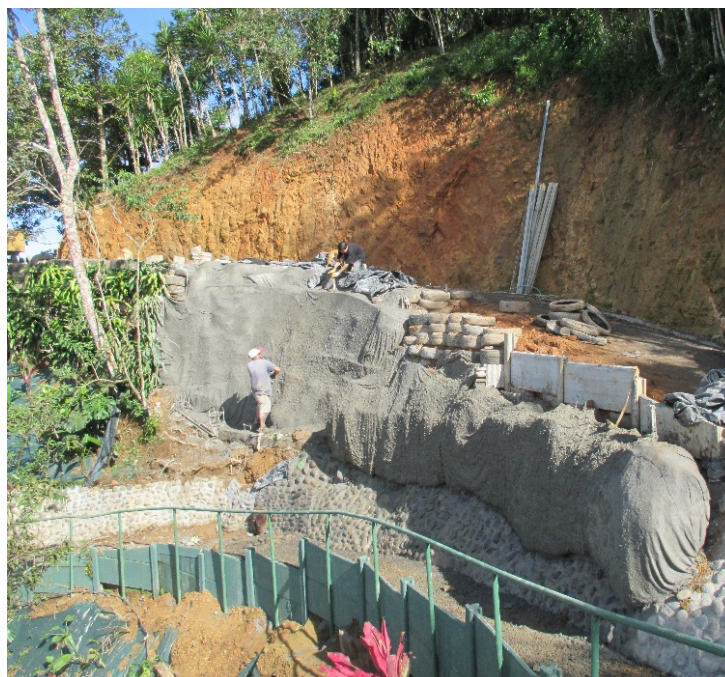
Stolen from Disney—Concrete-soaked material to cover the tire walls
