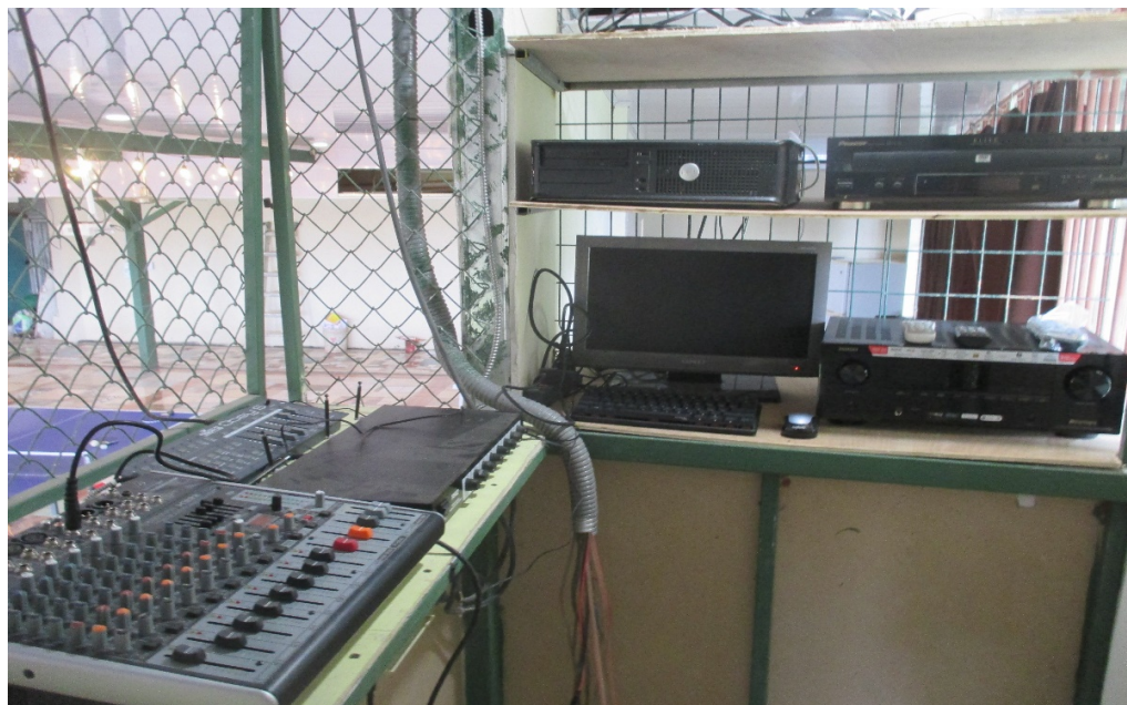
Activities Room Control Center
