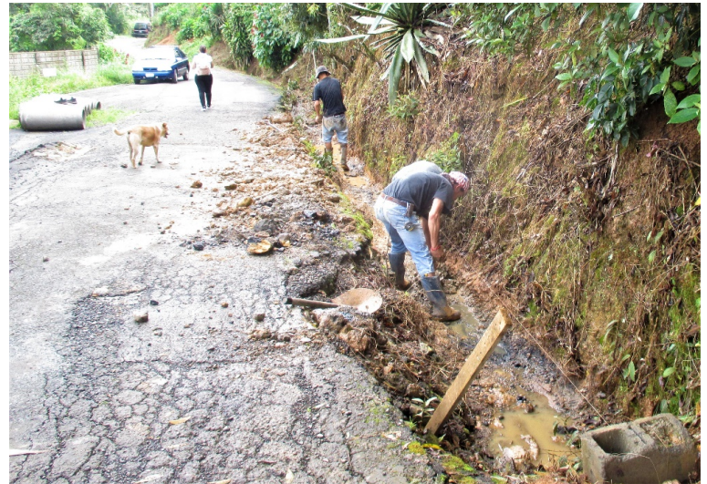
Left: lastre fill. Right: David Ugalde, JLT Work Foreman, leads the JLT work crew in culvert placement.
