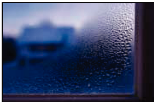
Condensation on the inside of a windowpane.
