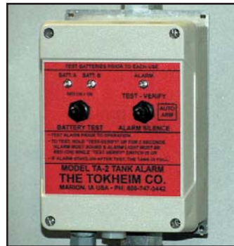
Top Left: TA-2 installed with a Tokheim No. 20 Tank Gauge.
