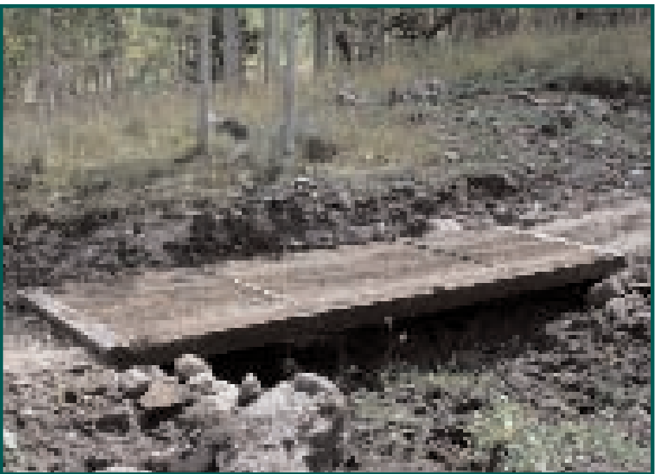
Harden or bridge stream crossings where appropriate to reduce sediment delivery.
