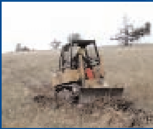
Mechanically constructed rolling dips or undulating trail grades provide water control and reduce maintenance.
