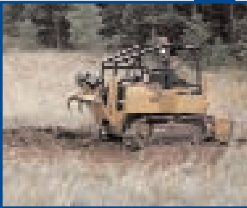
Mechanically constructed rolling dips or undulating trail grades provide water control and reduce maintenance.
