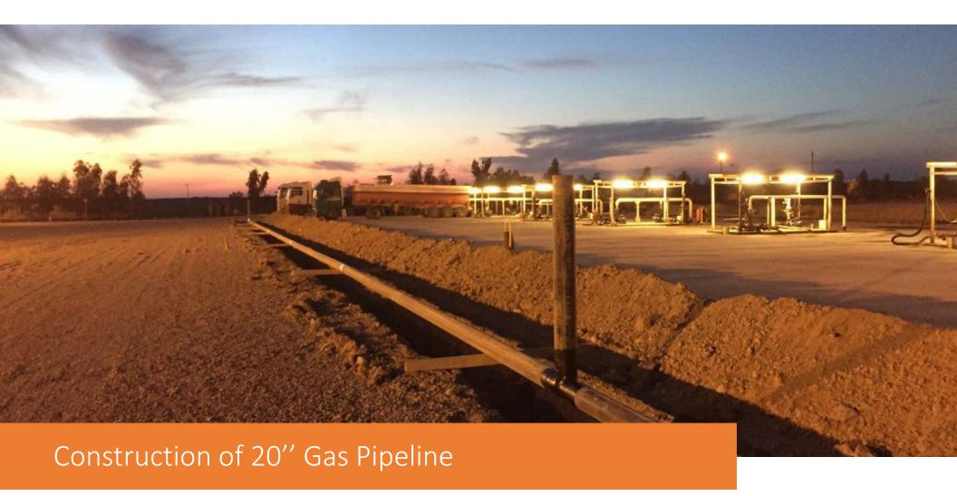
• **Description:** Right of Way (ROW), Stringing, Bending, Welding, Lowering, Casing / Road crossing, Tie-ins
