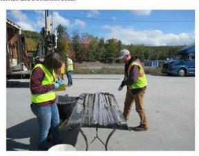
16.) View North – Groundwater Purge and Sampling of One (1") Inch *GeoProbe* Soil Boring Obtained for STARS 8260 / 8270 Laboratory Analysis.
