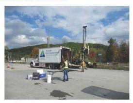
10.) View Northeast – Soil Coring to Approximately 20 Feet – Photo Depicts Soil Sample Boring and Groundwater Sampling Southwest and Downgradient of the Diesel Tank Area.
