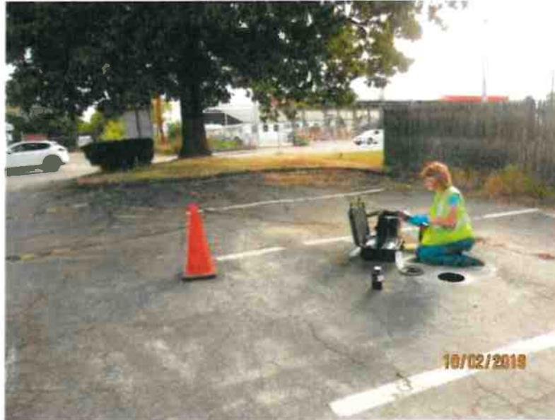
**10.) October 2, 2019:** Joseph Polsinello, LSP, IPC conducting initial elevation survey, phase layer assessment, confirmation of GW MW measurement, PID Headspace Screening, existing circa 1978, four (4") inch GW MW. Note: Well Located in the Central Area of the Asphalt Paved Parking Area.
