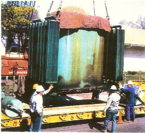
Removal of PCB Equipment from a High-rise Building.
