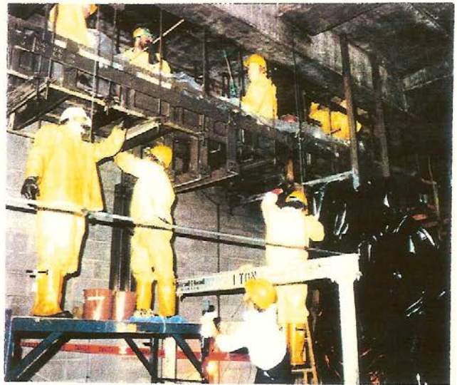
Removal of PCB Equipment from a High-rise Building.
