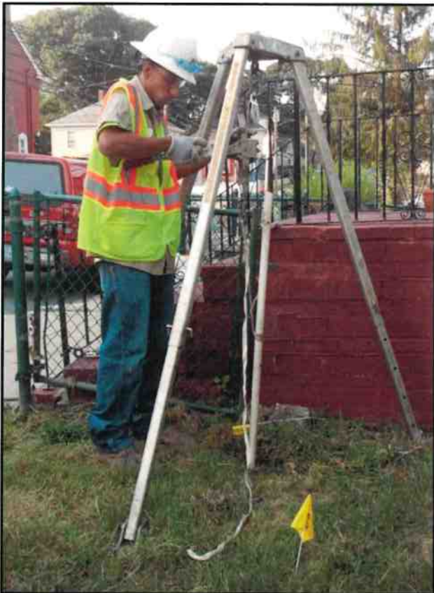
Pulling MW-2 on 9/3/15
