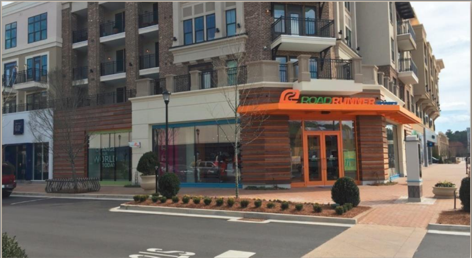
Commercial facade, Atlanta GA Thermo-treated Ash
