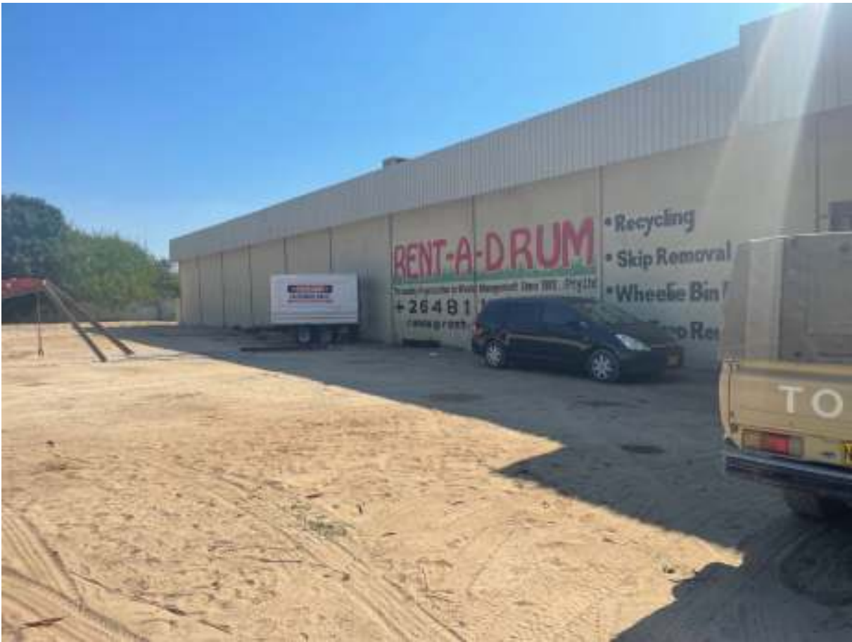
Plate 3.4: Rent-A-Drum waste management facility in Rundu (Marvin, 2021).
