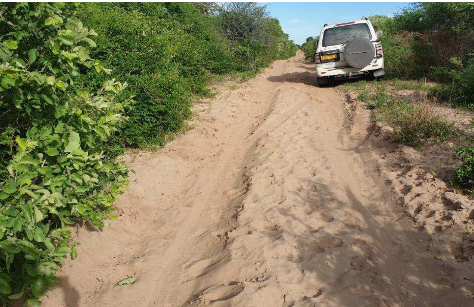
Plate 6.7: Local sandy tracks which might have localised compaction in some places creating a central ridge in the middle of the track which will make it difficult for lower raised vehicles to pass through the same tracks.
