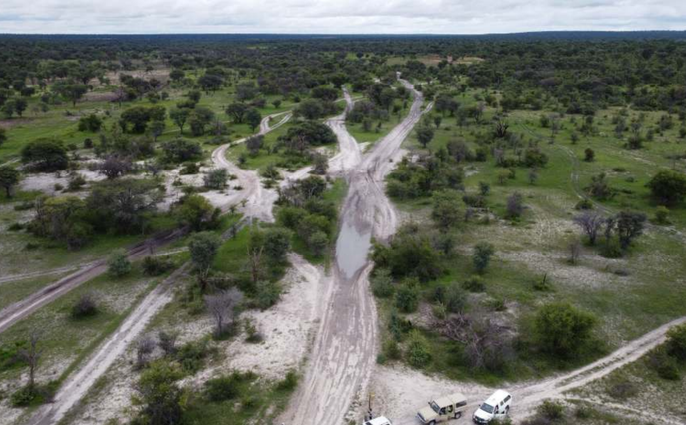
Plate 6.8: The poor conditions of the already damaged existing road from Ncaute to Naingopo. Existing roads and tracks will need to be upgraded before the start of drilling of the proposed prioritised D1-D6 and G1-G6 exploration and appraisal wells sites in the AOI within PEL No. 73.
