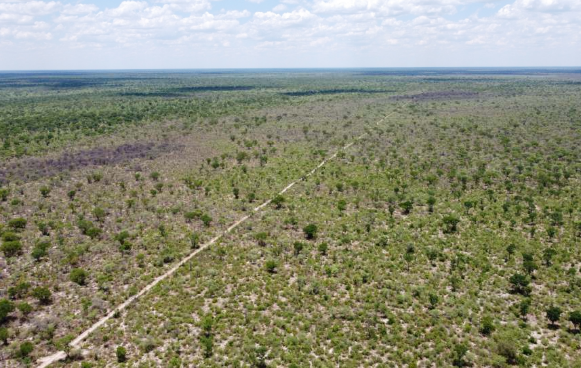
Plate 1.9: Drone image of the general surrounding area at the Damara Fold Belt Leads well location No. G6 and existing access.
