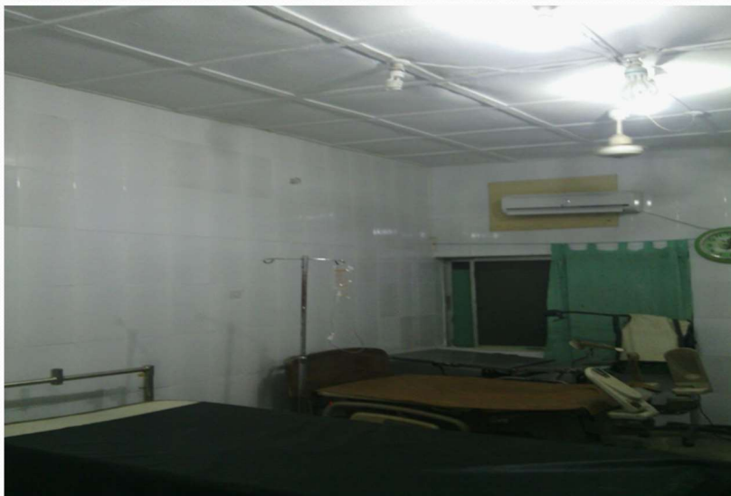
Renovated delivery suite, Umaru Sanda Ndayako General Hospital
