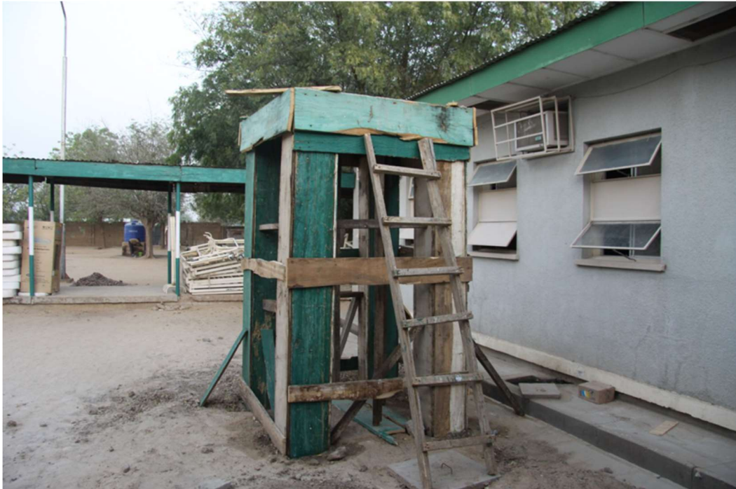
Overhead booster water tank stand for the delivery suite under construction
