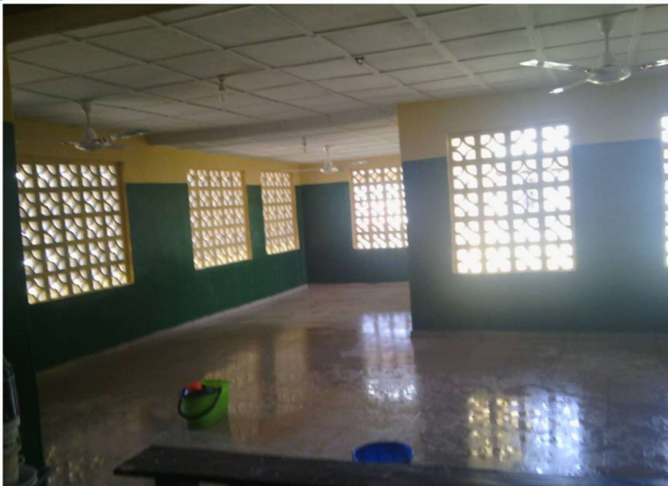
Completed Antenatal clinic at Umaru Sanda Ndayako General Hospital
