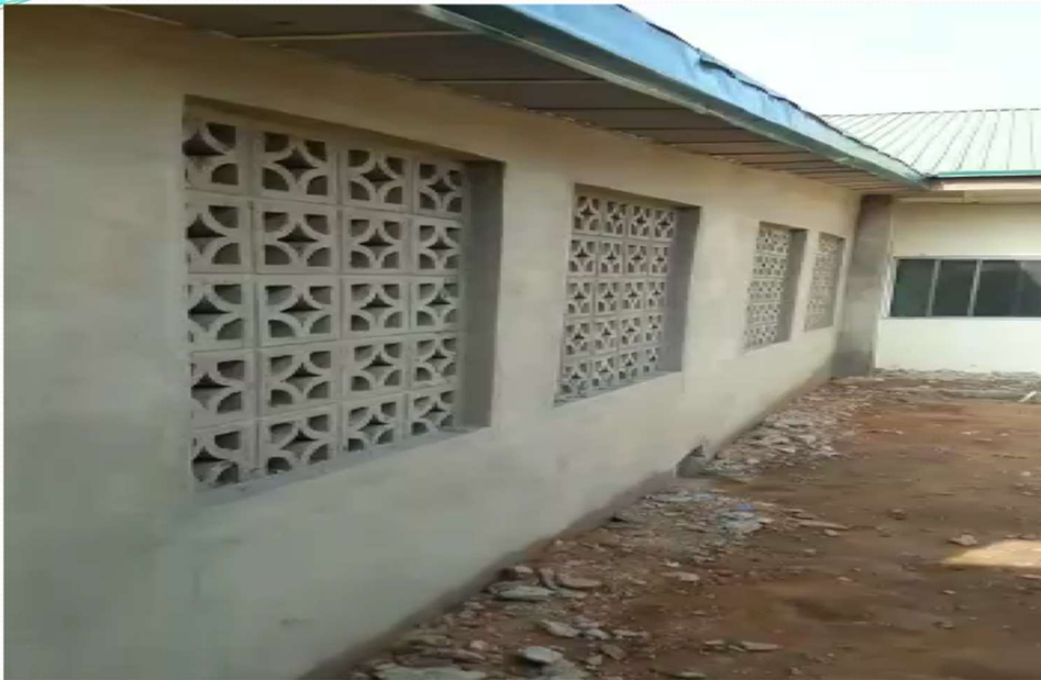
Completed Antenatal clinic at Umaru Sanda Ndayako General Hospital
