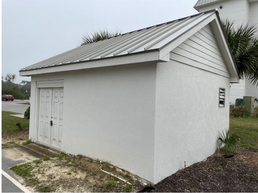
South and West Exterior
