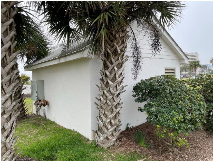
North and East Exterior
