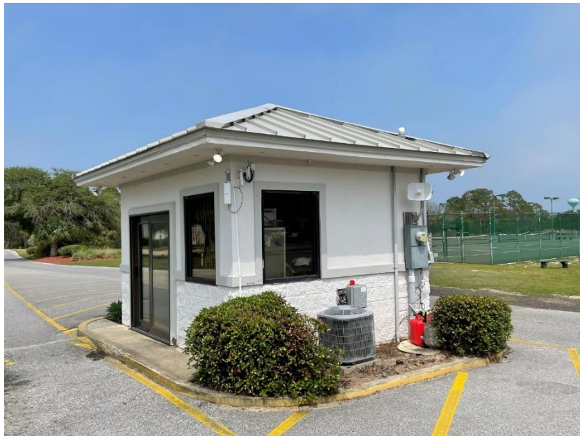
South and West Exterior
