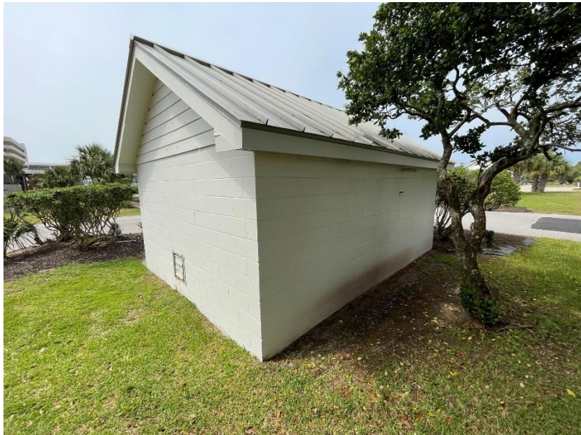
South and East Exterior
