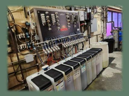
The SHAFT installed on a water feedline to a top-of-the-line chemical delivery panel
