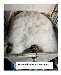
If the car wash uses chemistry manufactured with non-biodegradable surfactants or dyes, the biological treatments will fail to reduce dissolved solids and the use of a defoamer will be required to remove the foam load observed in the water tank.
