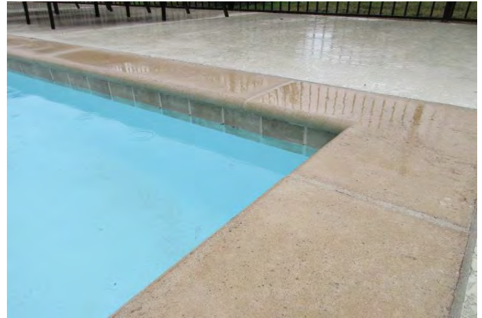
Tile scupper and concrete coping
