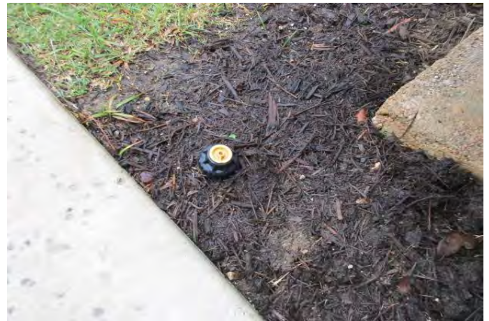
Irrigation system spray head
