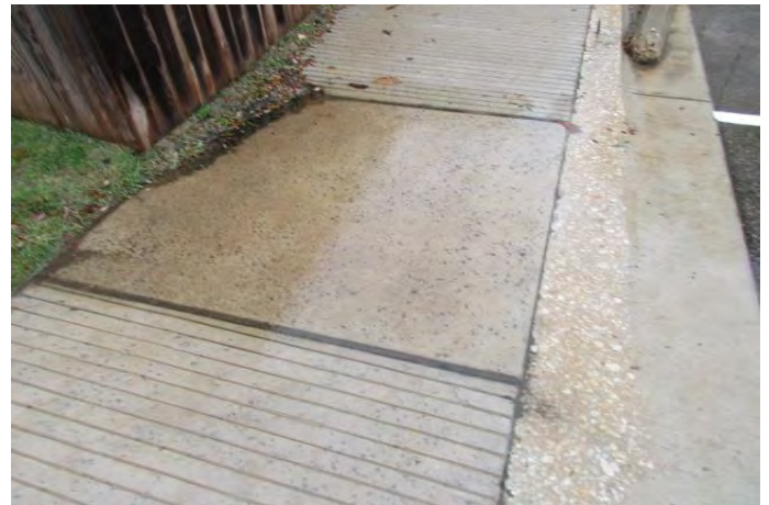
Low area at sidewalk that collects water
