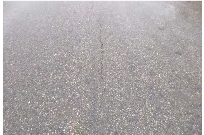
Small pavement crack
