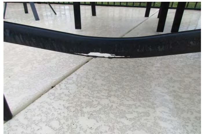
Finish deterioration at metal frame
