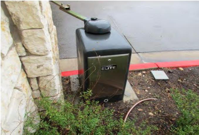
Swinging gate operator
