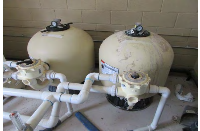
Filters, valves and piping
