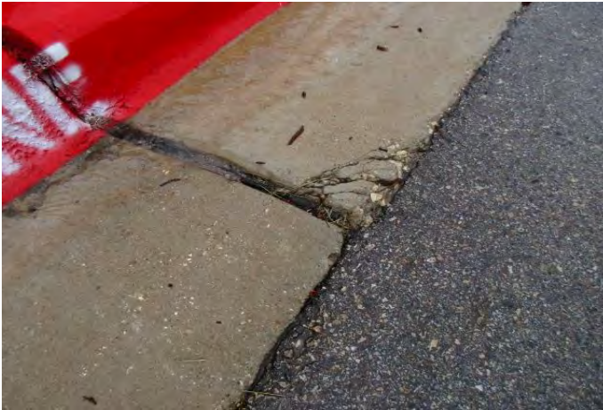
Cracked gutter
