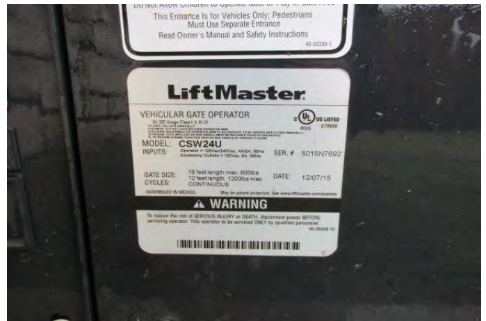
Gate operator name plate
