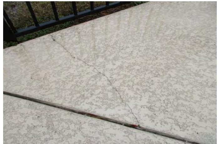
Crack at pool deck coating
