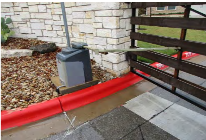
Swinging gate operator
