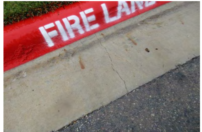
Cracked gutter
