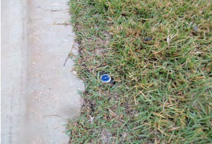
Irrigation system spray head
