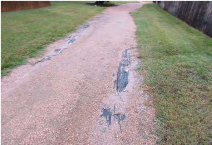
Eroded decomposed granite
