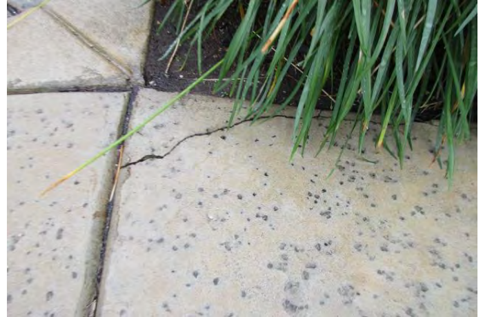
Cracked and spalled concrete sidewalk
