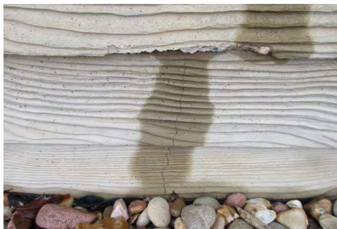
Crack at wall
