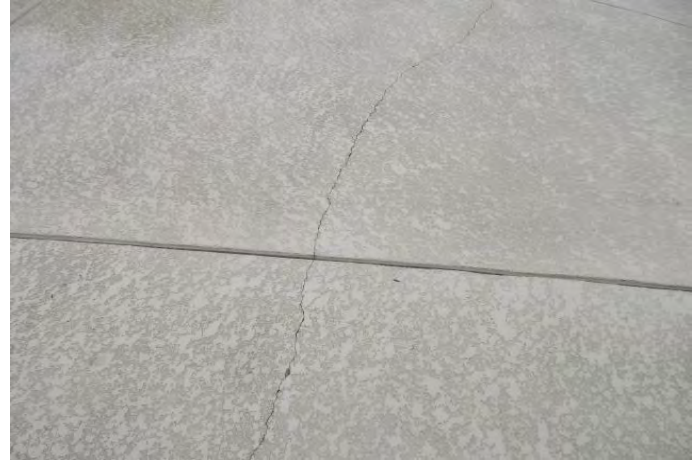
Pool deck coating crack
