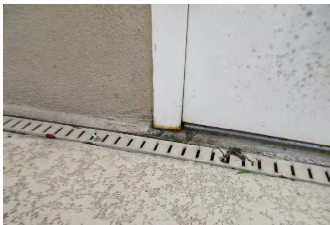
Rust at metal door frame
