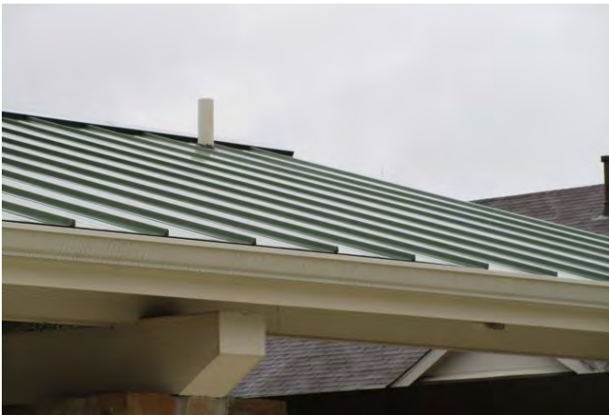
Standing seam metal roof
