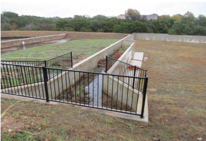
Concrete retaining walls
