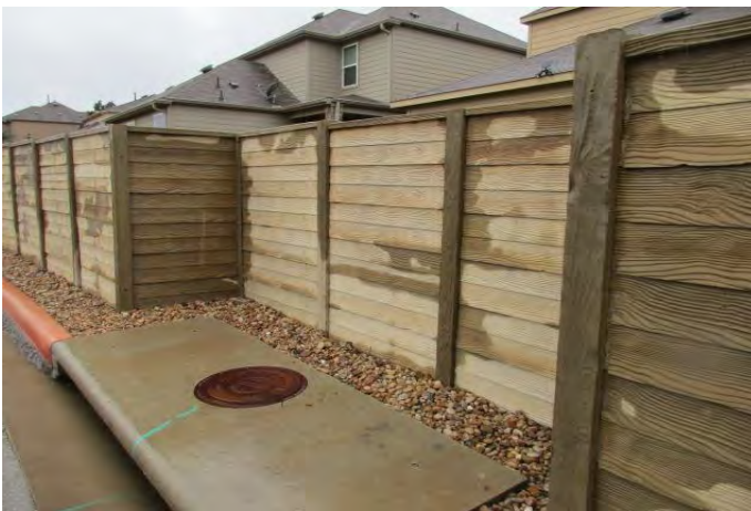
Concrete perimeter wall
