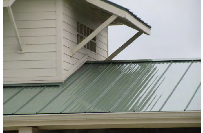
Standing seam metal roof
