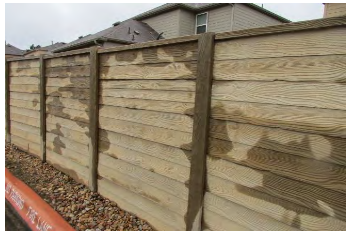
Concrete perimeter wall
