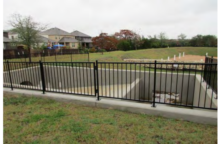
Fencing at storm water management feature
