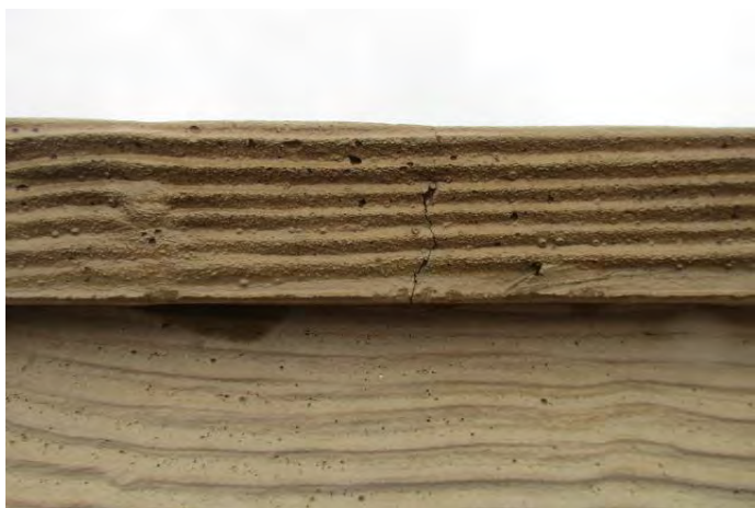
Crack at wall
