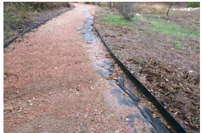
Erosion at path
