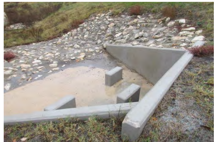
Water outflow structure
