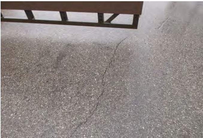
Small pavement crack
