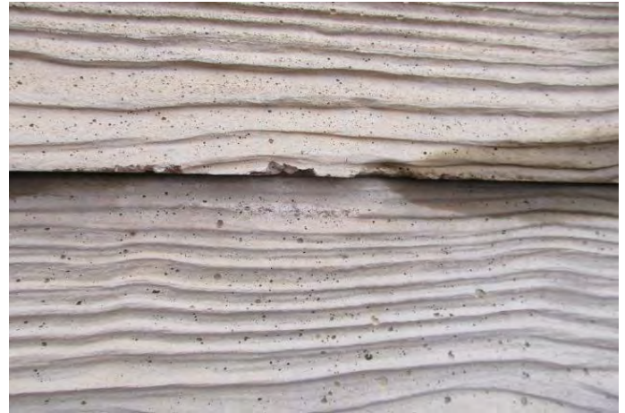
Deterioration of panel edge
