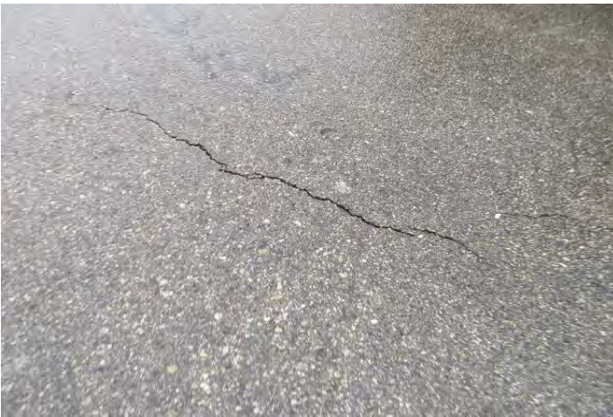
Small pavement crack
