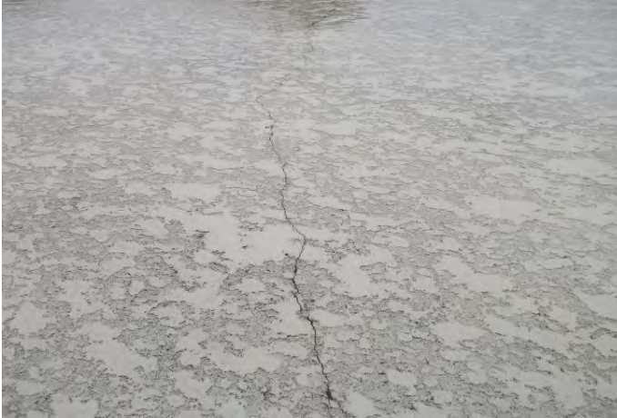
Crack at pool deck coating
