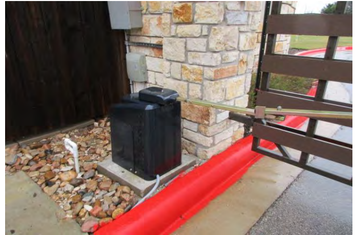
Swinging gate operator
