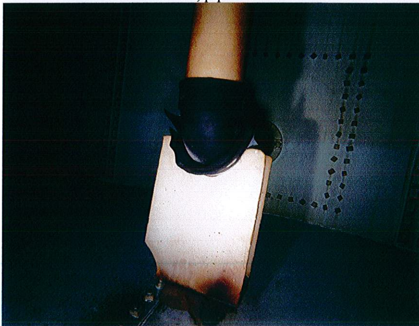
Bottom of overflow supported by a rock
