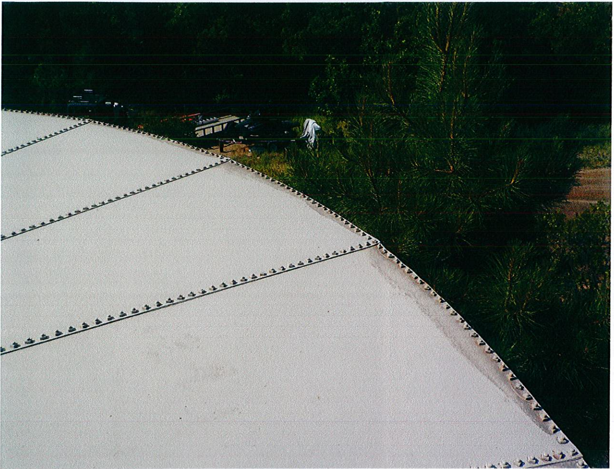
The roof is in good condition, no rust or peeling paint.
