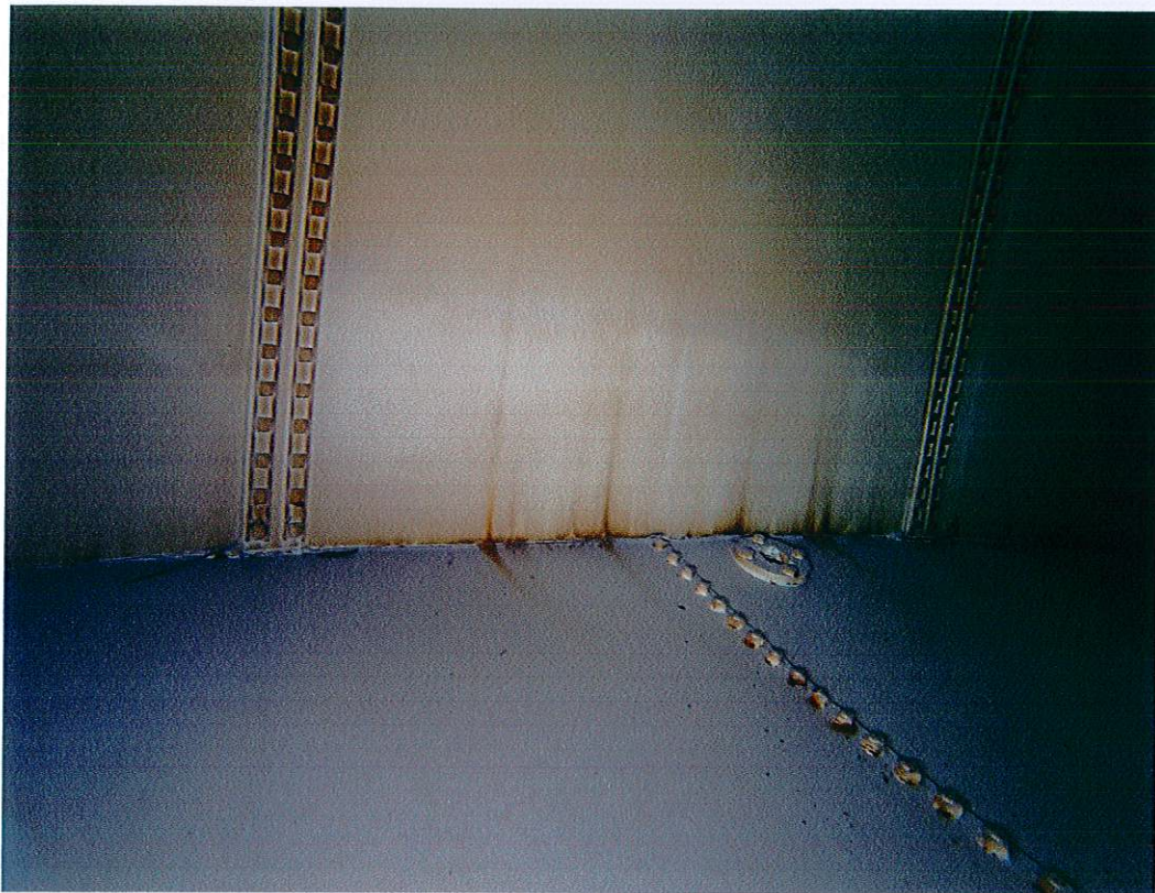
Minor corrosion at floor/shell area. Drain on floor.
