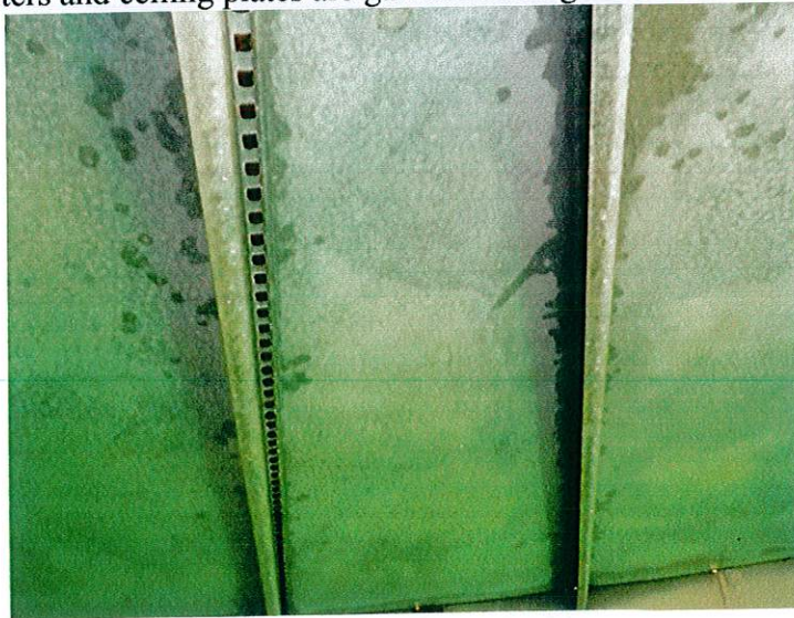
Rafters and ceiling plates are galvanized in good condition
