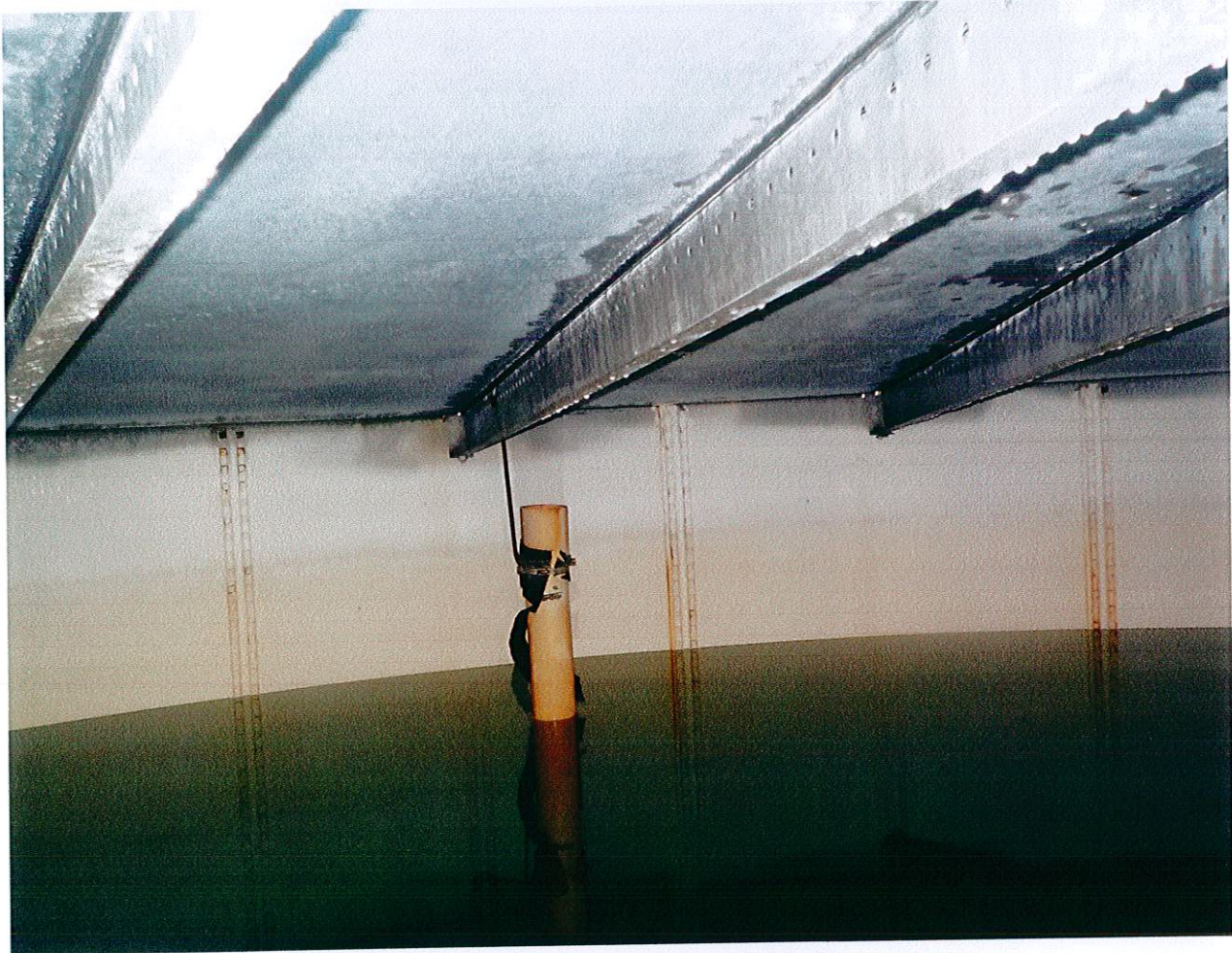
Rafters and ceiling plates are galvanized in good condition
