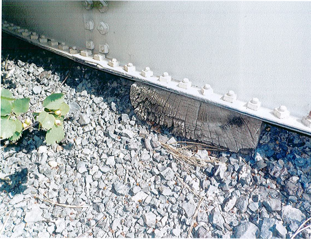
Wood skids for floor support
