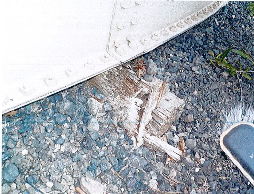
Wood skids for floor support
