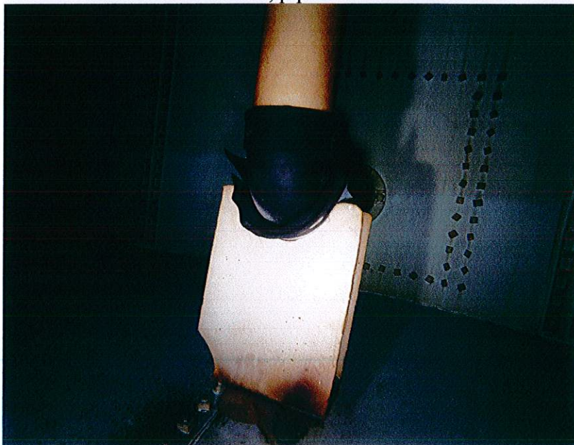
Bottom of overflow supported by a rock
