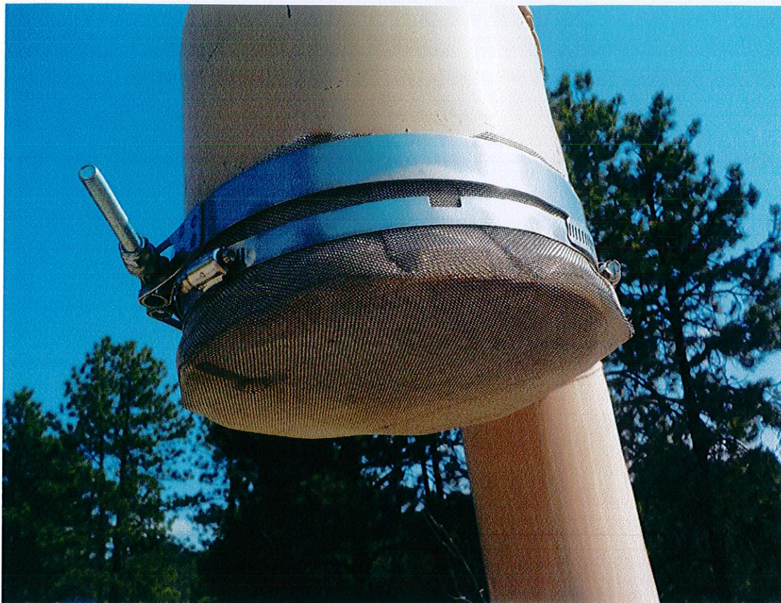
Vent screen is in place, securely fastened.
