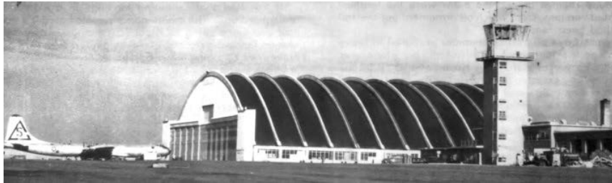
Rapid City Air Force Base B-36 Hangar, 1952
