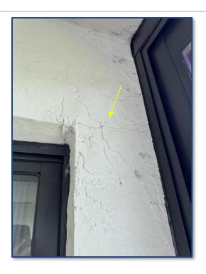
Photograph No. 19: Unit 108: Wall cracking observed near unit sliding glass door.
