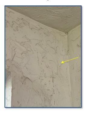
Photograph No. 24: Unit 101: Wall cracking observed near unit sliding glass door.
