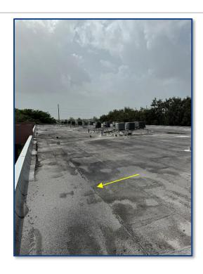
Photograph No. 31: Debris buildup from previous ponding water observed.
