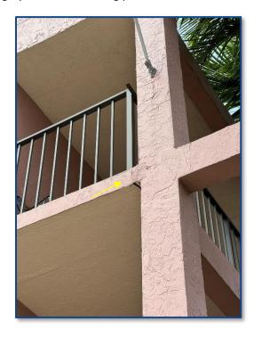
Photograph No. 10: Deteriorated expansion joint observed at 3<sup>rd</sup> floor near elevator.
