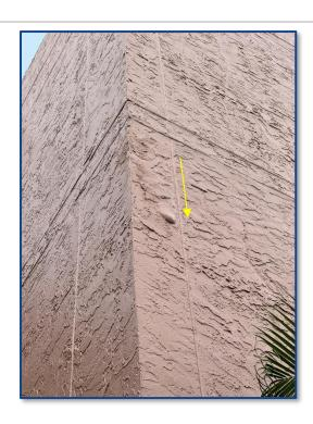
Photograph No. 9: Blistering paint observed at building edge.
