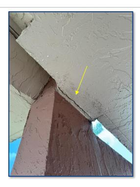
Photograph No. 11: Deteriorated expansion joint observed at 3<sup>rd</sup> floor near elevator.
