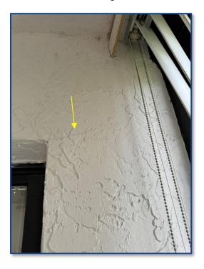
Photograph No. 20: Unit 106: Wall cracking observed near unit sliding glass door.
