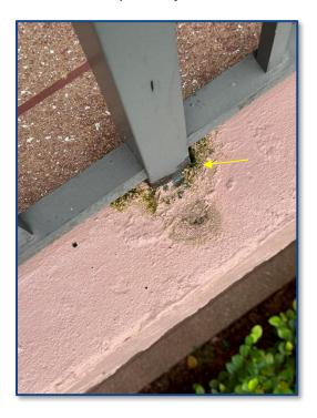
Photograph No. 12: Deteriorated railing post pocket observed near unit 208.
