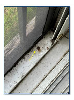
Photograph No. 27: Unit 205: Deteriorated fasteners observed at aluminum enclosure bottom rail.
