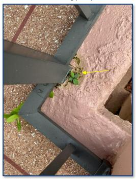
Photograph No. 14: Deteriorated railing post pocket observed near unit 208.
