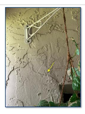
Photograph No. 23: Unit 101: Wall cracking observed near unit sliding glass door.
