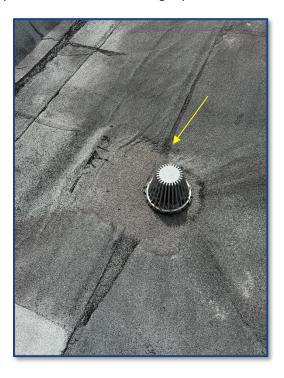
Photograph No. 30: Debris buildup near roof drain.
