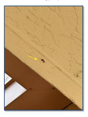
Photograph No. 18: Rust spot observed overhead near unit 310.
