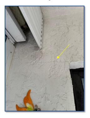
Photograph No. 22: Unit 103: Wall cracking observed near unit sliding glass door..
