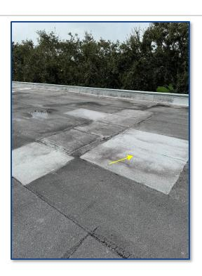
Photograph No. 29: Previous roofing repairs observed at the roof.
