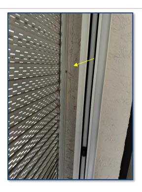
Photograph No. 25: Unit 205: Wall cracking observed near balcony enclosure.
