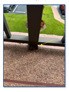
Photograph No. 16: Deteriorated railing post pocket observed near unit 310.
