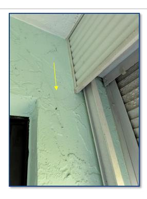
Photograph No. 21: Unit 104: Wall cracking observed near unit sliding glass door.
