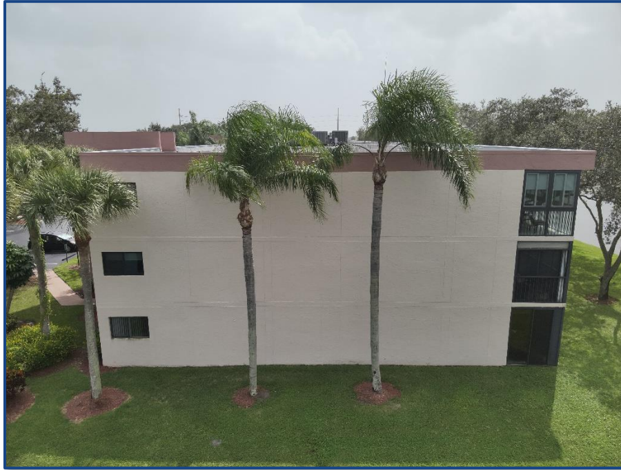
Photograph No. 1: Building North Elevation
