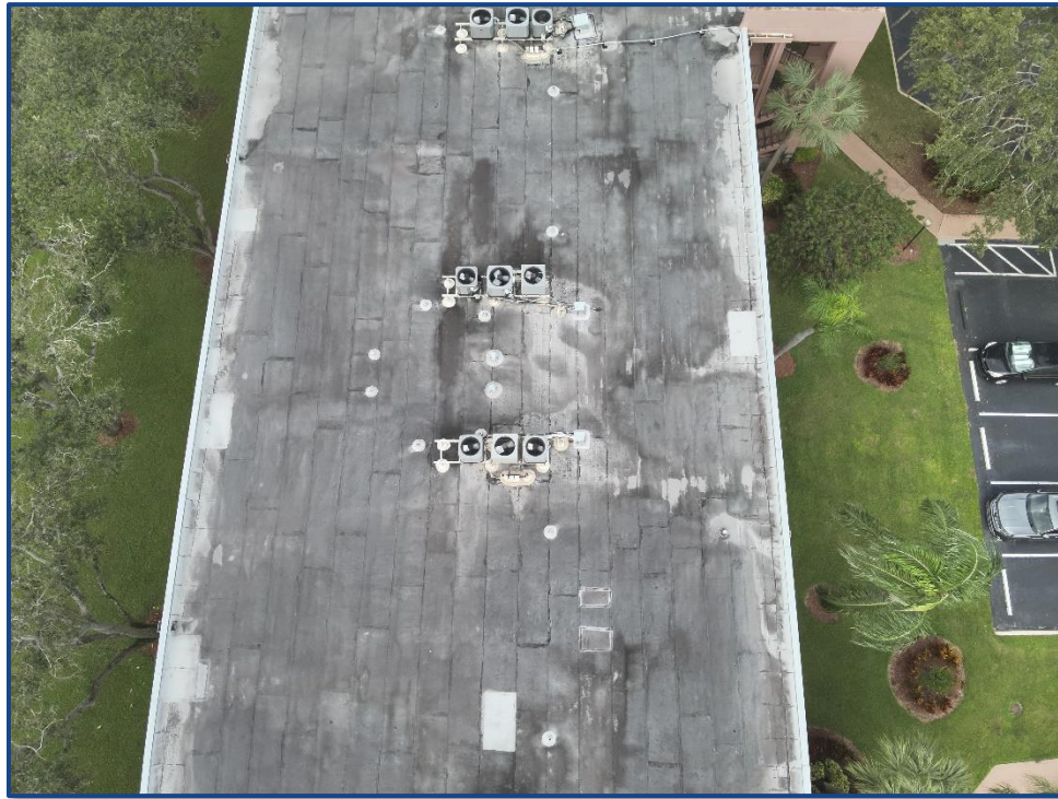
Photograph No. 5: Building Roof
