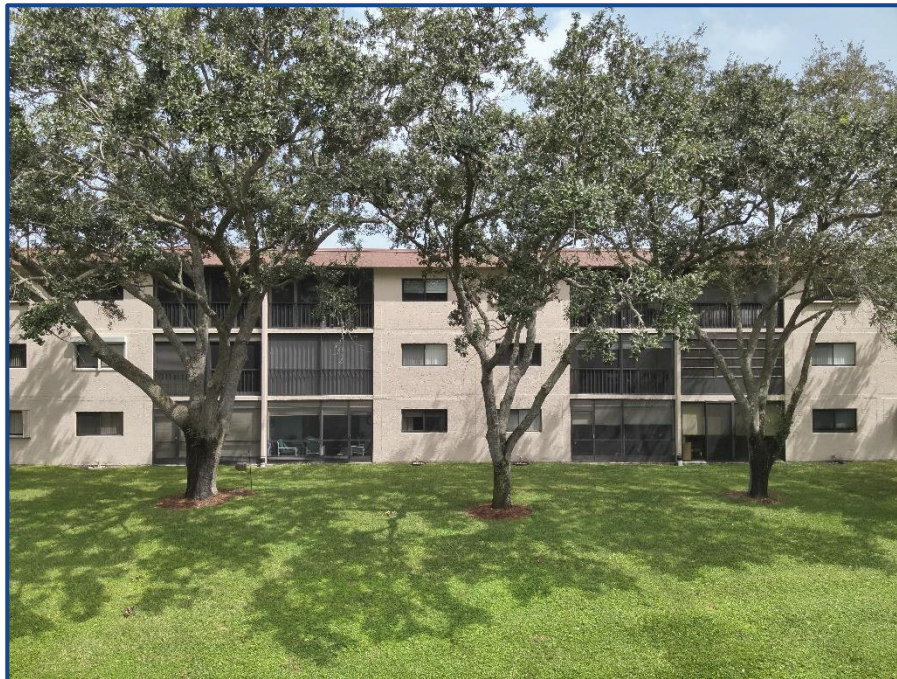
Photograph No. 2: Building Typical West Elevation
