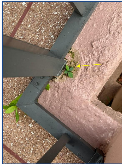
Photograph No. 13: Deteriorated railing post pocket observed near unit 208.
