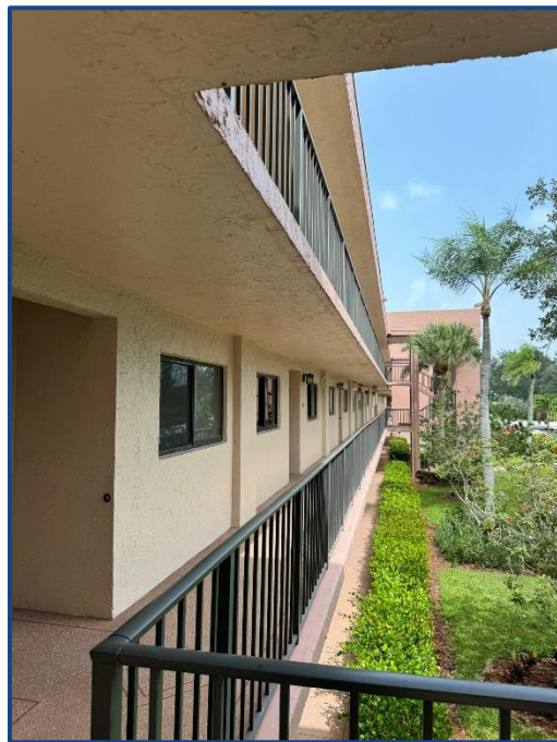
Photograph No. 8: Typical Building Catwalk
