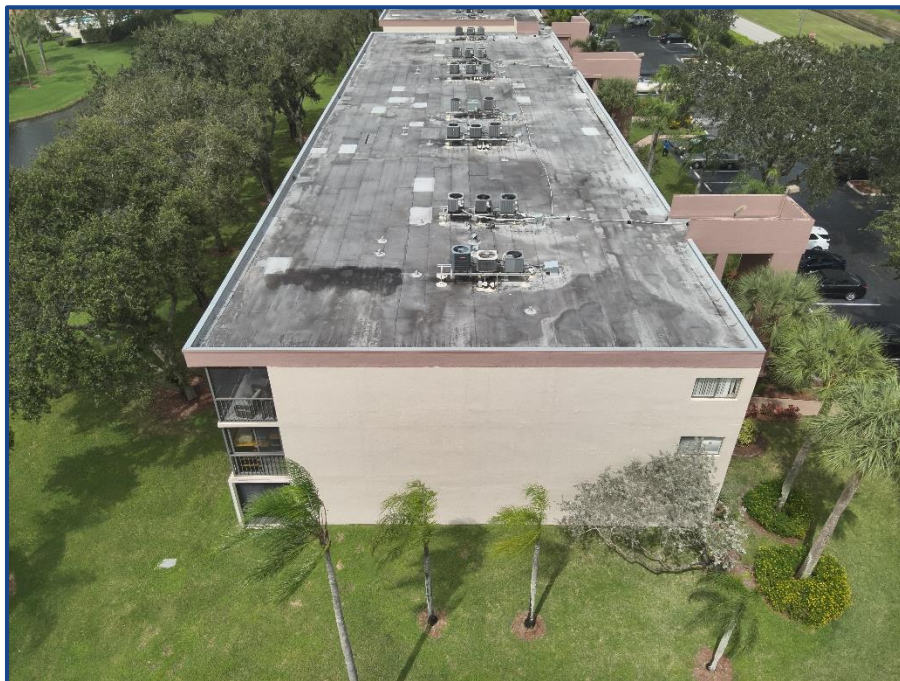
Photograph No. 4: Building South Elevation
