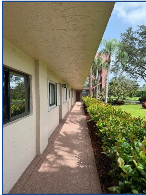
Photograph No. 7: Typical Building Catwalk
