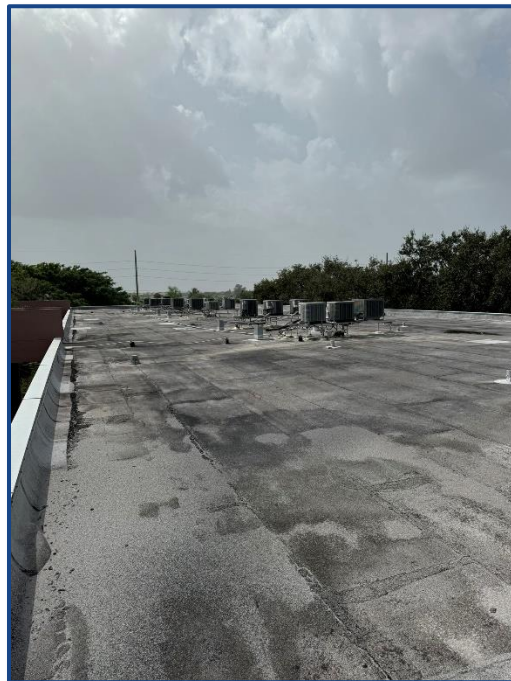
Photograph No. 6: Building Roof
