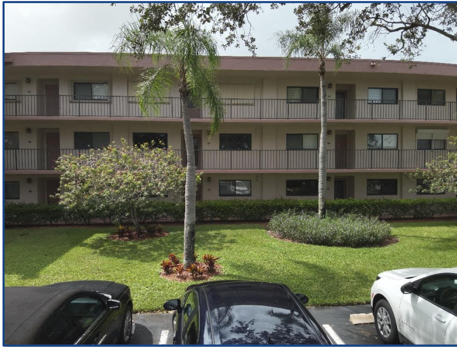
Photograph No. 3: Building Typical East Elevation
