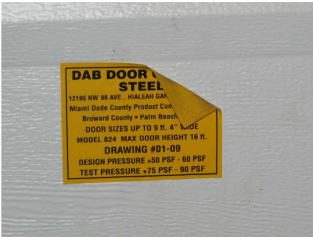
Impact rated garage door label (located on the inside)
