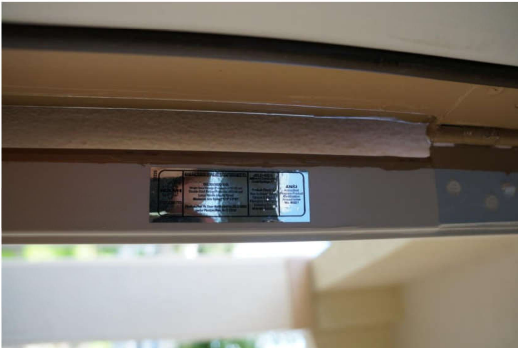
Impact rated door label on its typical location
