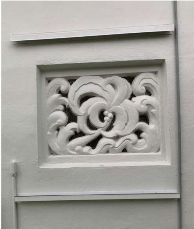
Decorative masonry/stucco opening with impact protection
