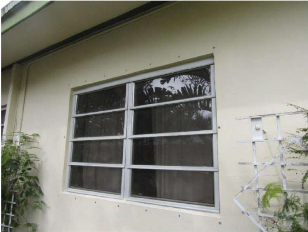
Window anchors directly on wall for hurricane panels (check building codes, anchors may need to be drilled every 6 inches)
