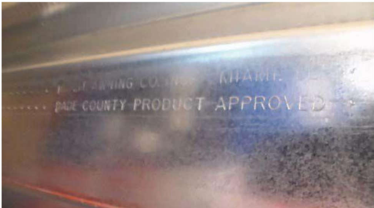
Engraving on shutters/panels - county approved product
