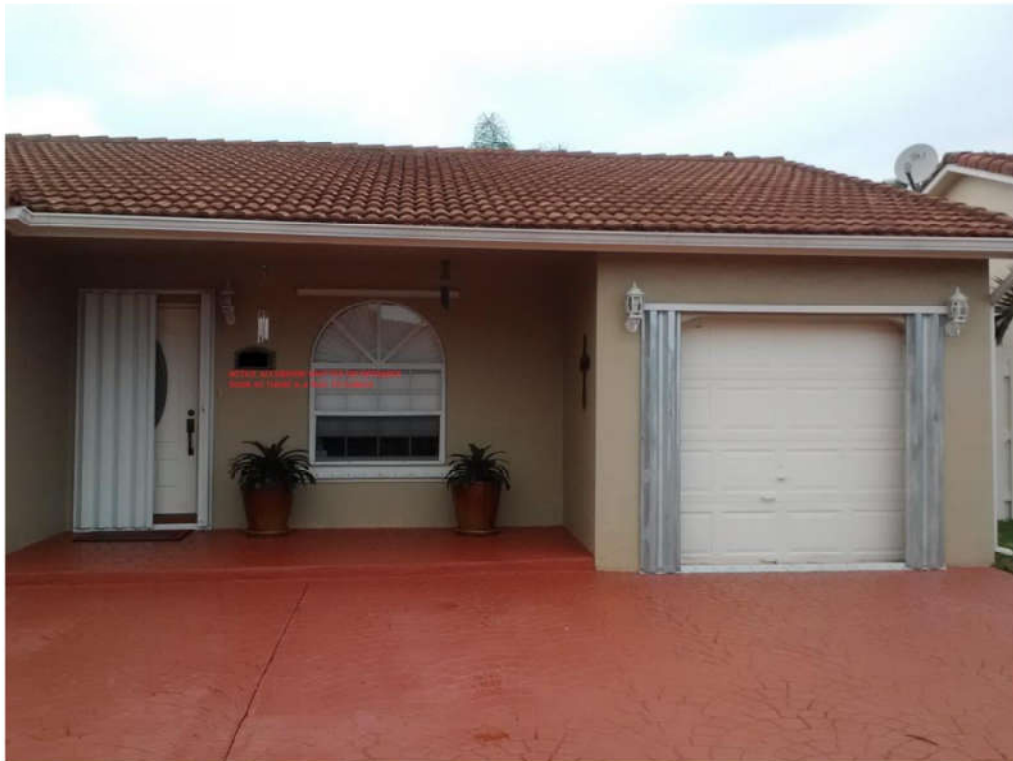
Alternative way of protecting garage door (and front door) when it is not impact rated
