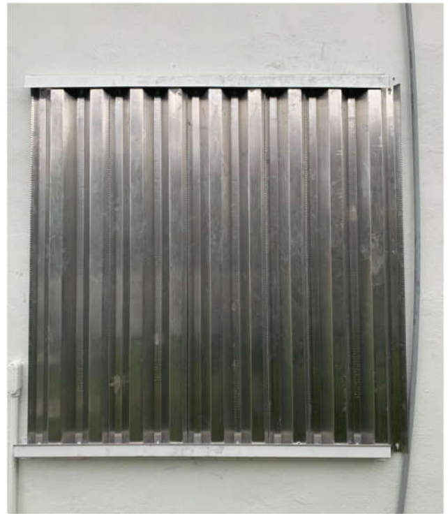
Decorative masonry/stucco opening with impact protection
