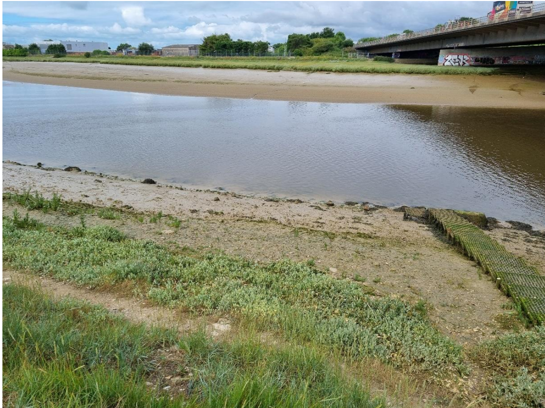
Figure 18 Unofficially access point near the Adur Flyover showing a raised path to the channel.
