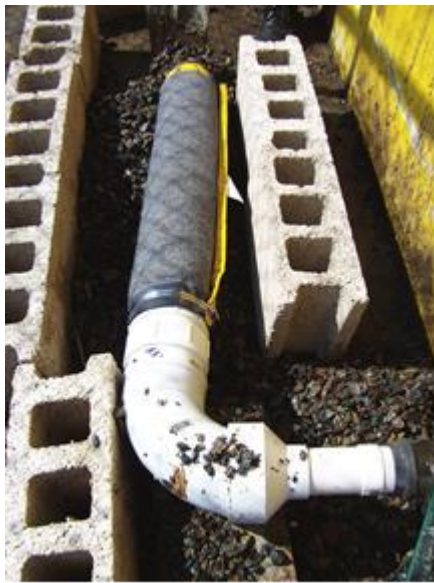
Pad Mount Install
