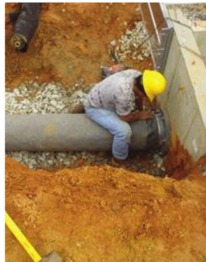
Water Gate Install
