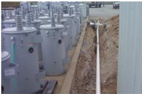
Pad Mount Install
