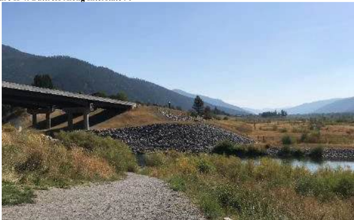
Figure H-4: Buttress Along Interstate 90
