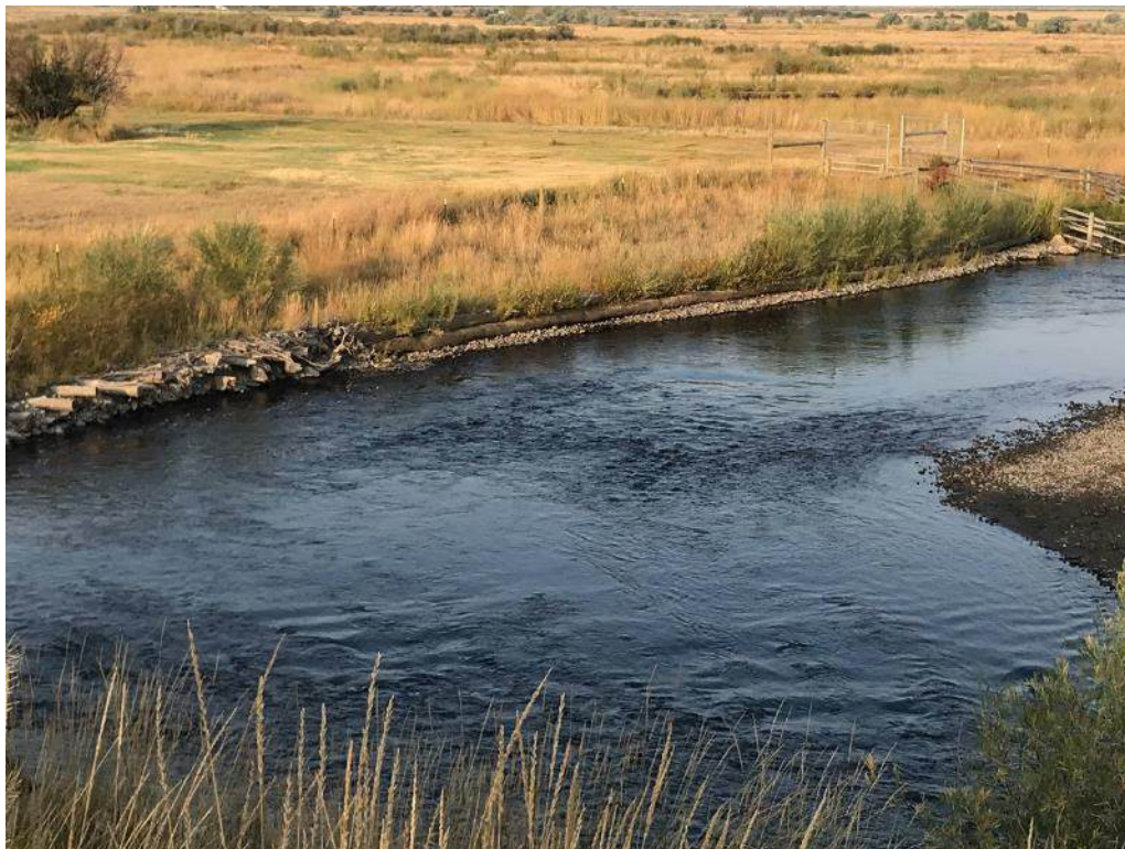
Figure H-15: Bank Stabilization on Clark Fork River with Sediment Deposition on Inside Curve
