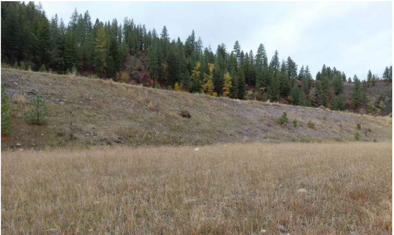
Side slope of Tunnel Pond Repository
