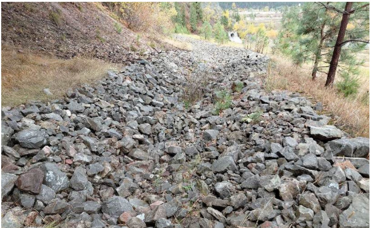
Drainage channel at the top of Tunnel Pond Repository
