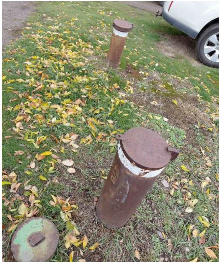
Monitoring wells MW-99A and MW-99B, which were not secured
