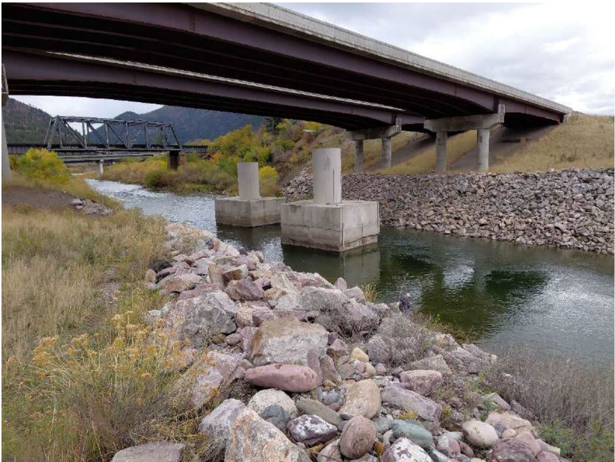
Rip-rap along Blackfoot River under I-90 overpass, unused pylons in the center of the river (expected to be removed), railroad bridge in the background, looking Northeast
