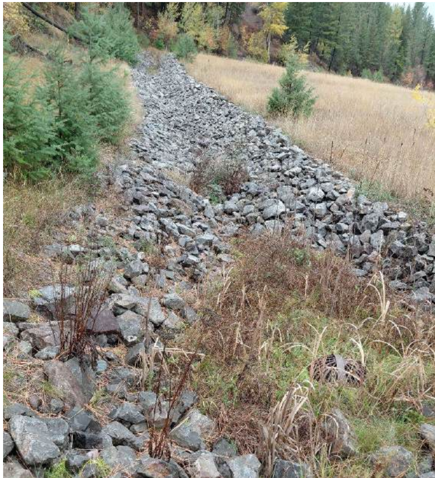
Surface water drainage channel and drop structure
