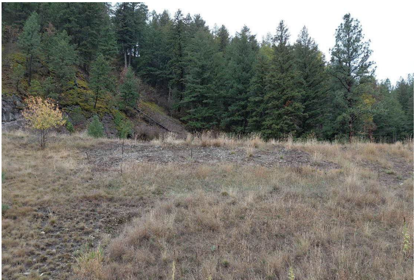
Bare area on Tunnel Pond Repository side slope
