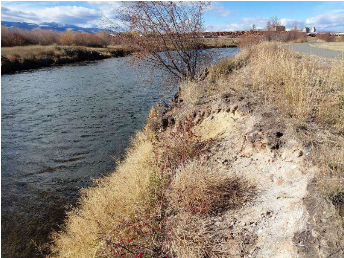
Streambank erosion along the Clark Fork River in Arrowstone Park. Note yellow soil indicating possible tailings.
