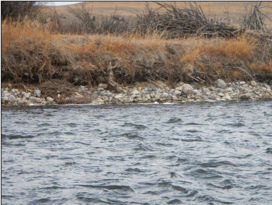
**Figure 2-70. Cobble toe in left bank, Subreach A7, Phase 20, RM 41.5.**
