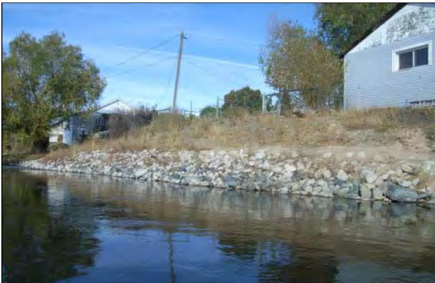
Figure 2-60. Rock riprap bank armor, Subreach A5, Phase 14, RM 29.4.
