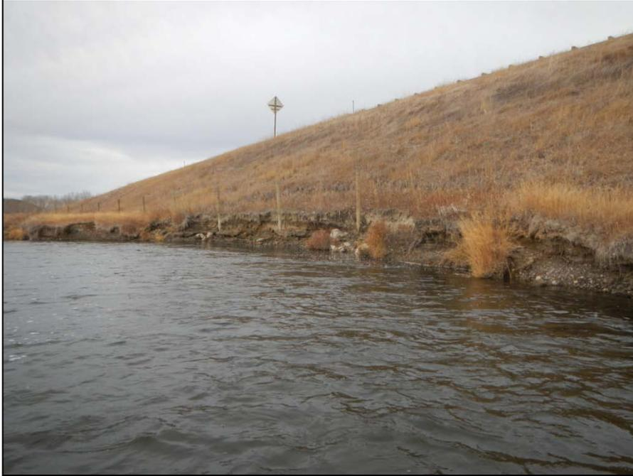
Figure 2-76. View downstream of erosion into I-90 embankment, Subreach A7, Phase 22, RM 42.25.
