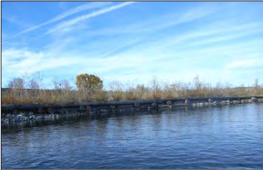
Figure 2-59. Left bank cribwall bank protection Subreach A5, Phase 14, RM 29.4.
