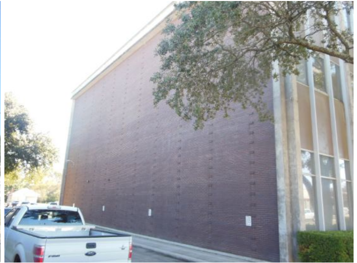
Left Side - Brick Exterior
