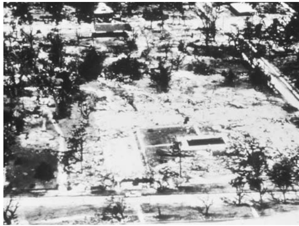
Two of the most famous photographs in the study of tropical cyclones, these before-and-after photographs of the Richelieu Manor apartment building in Pass Christian, Mississippi, are often held as an example of the unmitigated destructive potential of intense hurricanes. The Richelieu’s Gulfside location made it an unhappy target for Camille’s 25-foot (8-m) storm surge. (NOAA)
