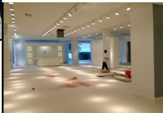
Pre-/Post Construction Clean Up
