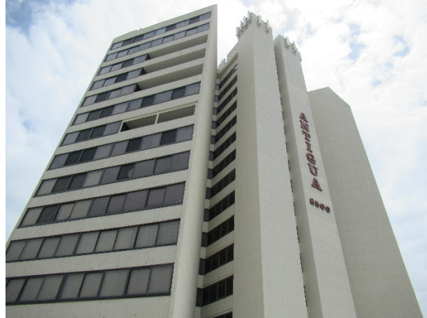
Exterior stucco walls overview
