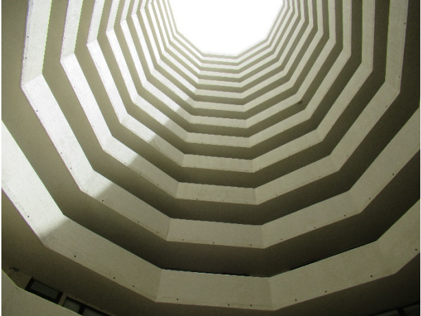
Interior stucco walls overview
