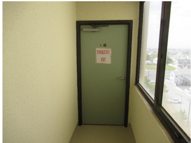
Typical unit door
