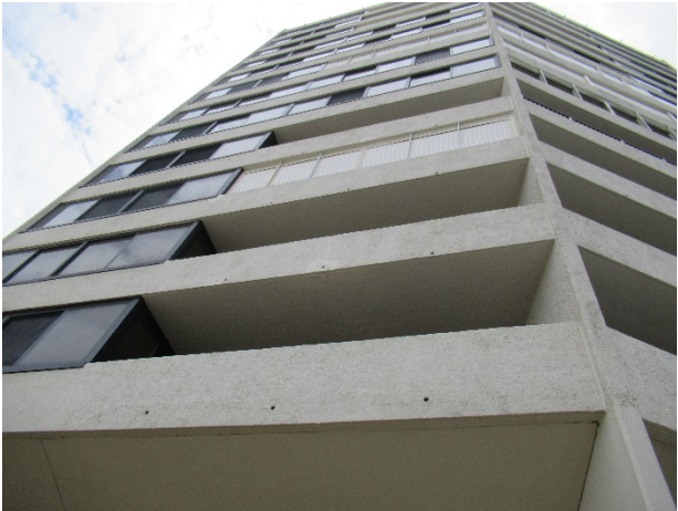
Typical exterior balconies
