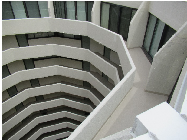
Interior balcony overview (14 th floor only)
