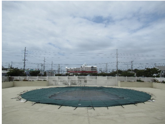
Pool area overview
