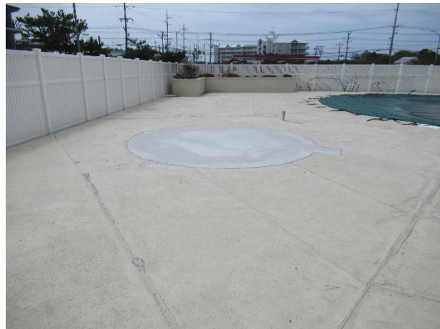
Pool deck overview and filled in structure
