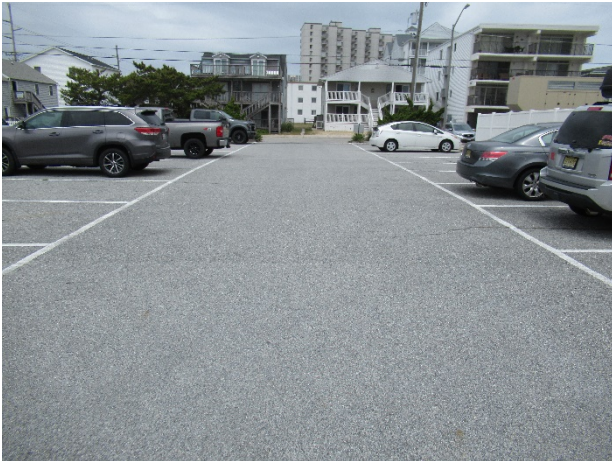
Asphalt pavement parking area overview
