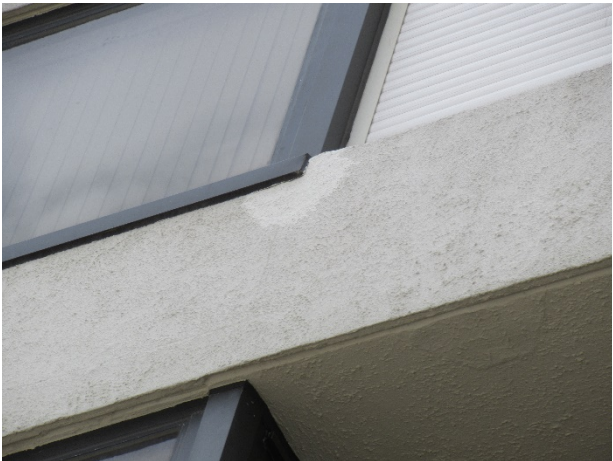
Previous stucco repair at window
