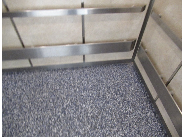
Elevator cab finishes
