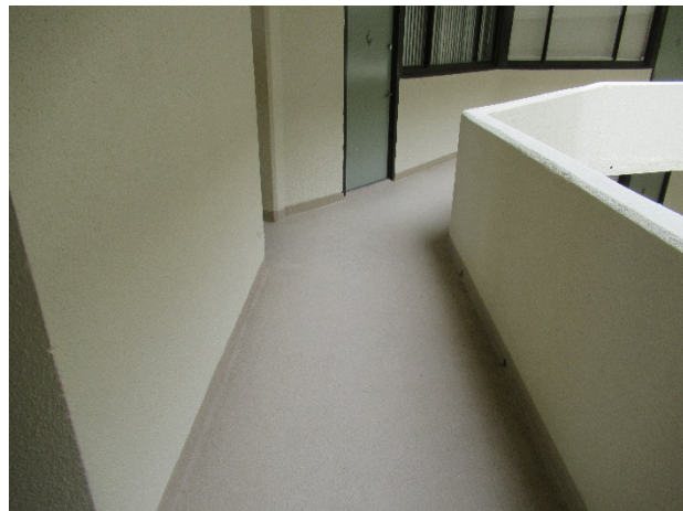
Interior walkway surface
