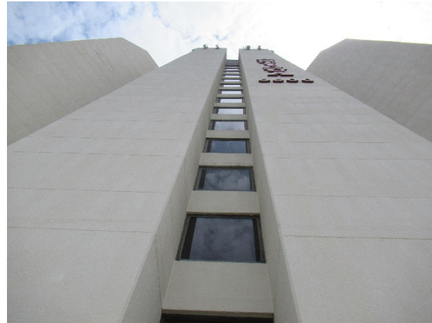
Elevator lobby windows overview
