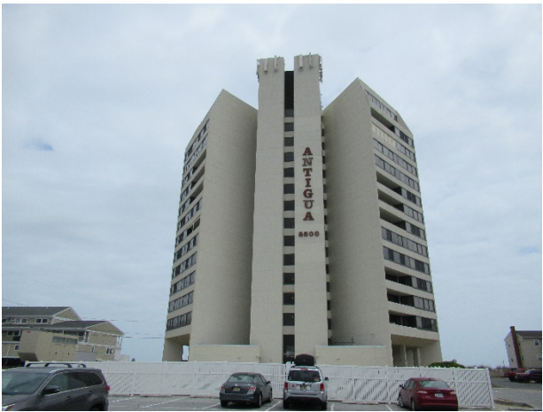
Front elevation overview
