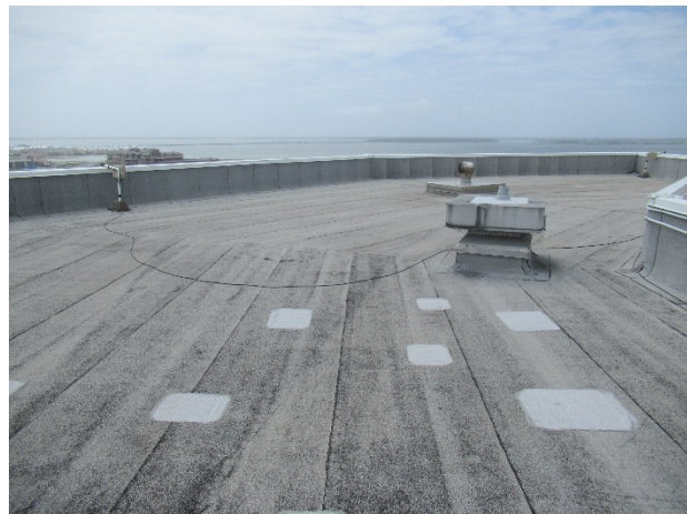
Previous roof repairs
