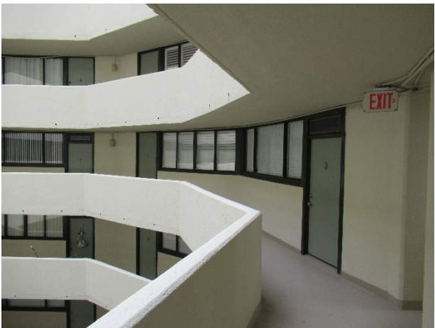
Typical interior walkway overview
