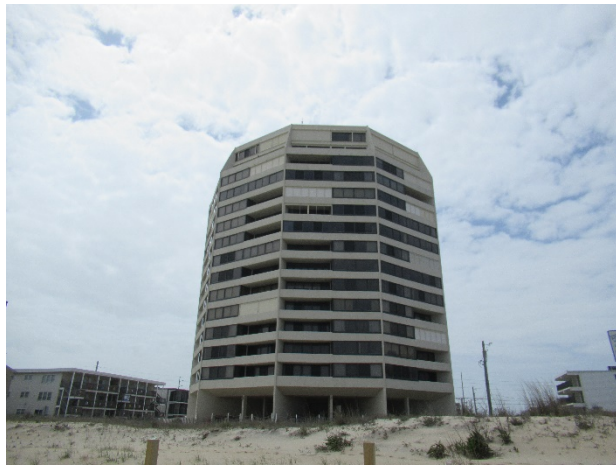
Rear elevation overview
