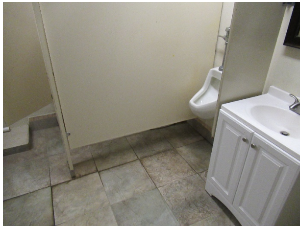
Rest room floor covering, partition and plumbing fixture overview
