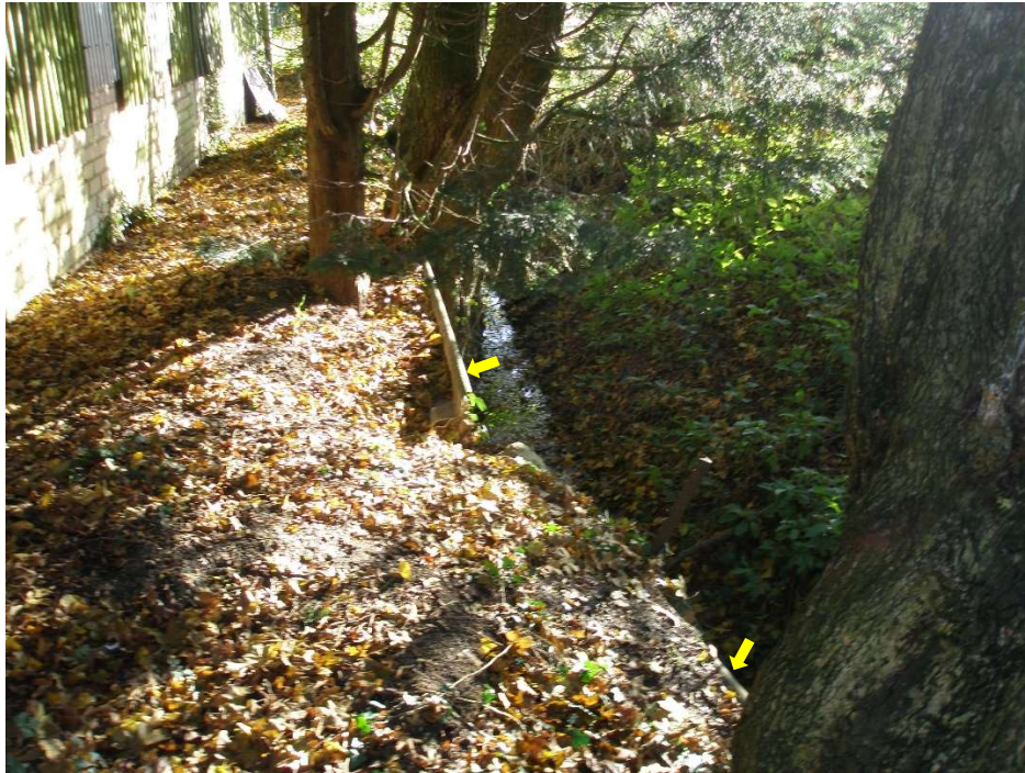
Southern boundary drain. Arrows show positions of cement sheet (possible ACMs) supporting bank
