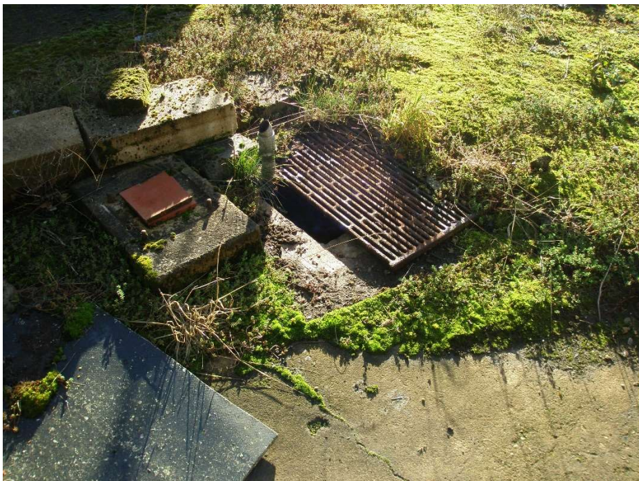
Riser pipe for historic abstraction borehole operational between 1948 and mid-60s
